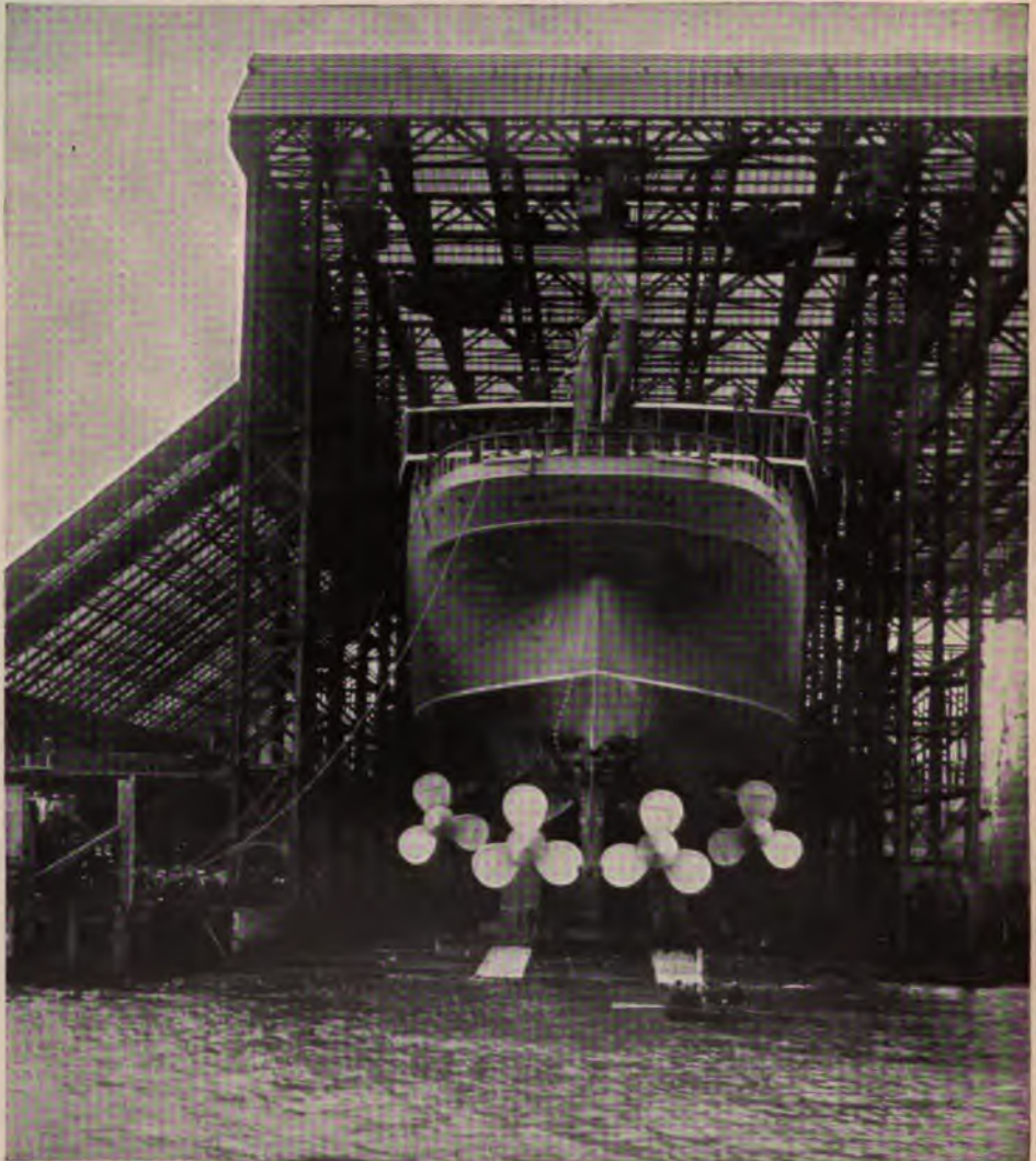
FIG. 60.—Stern View of 'Mauretania' before Launching.
