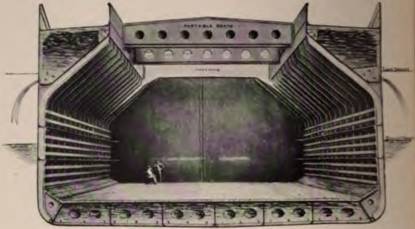
Hold View of Cantilever Framed Ship, Single-Deck Type.
