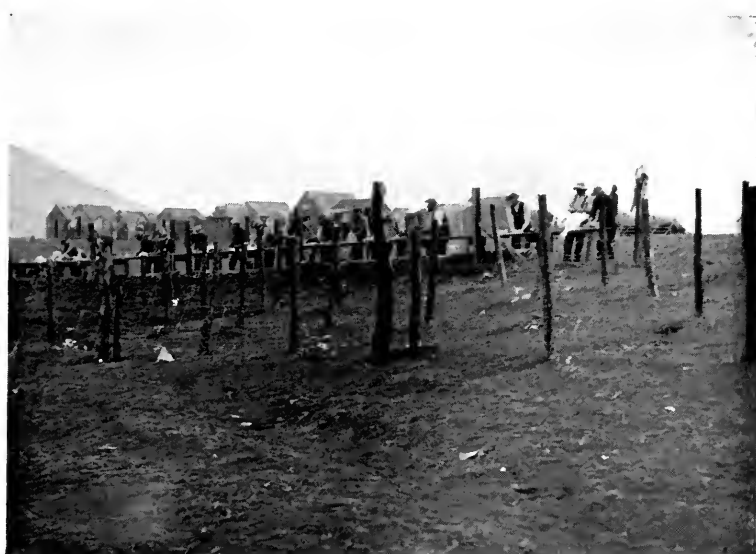
SCENE IN CAMP, WASHING DAY. (Showing Barbed Wire Fencing.)
