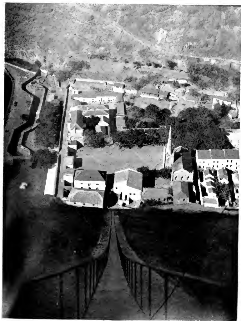
JAMESTOWN FROM TOP OF THE LADDER (LOOKING DOWN).
