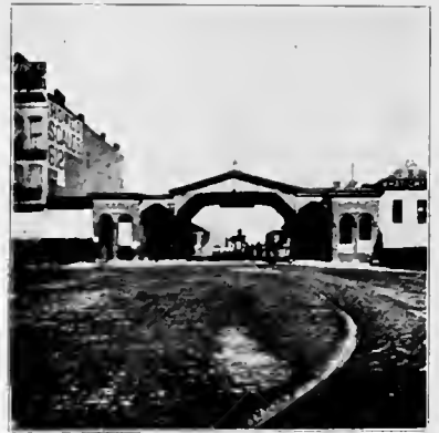
ORIGINAL ENTRANCE TO THE EADS BRIDGE
