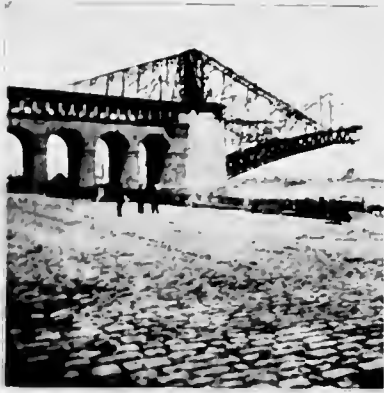
EADS BRIDGE IN COURSE OF CONSTRUCTION
