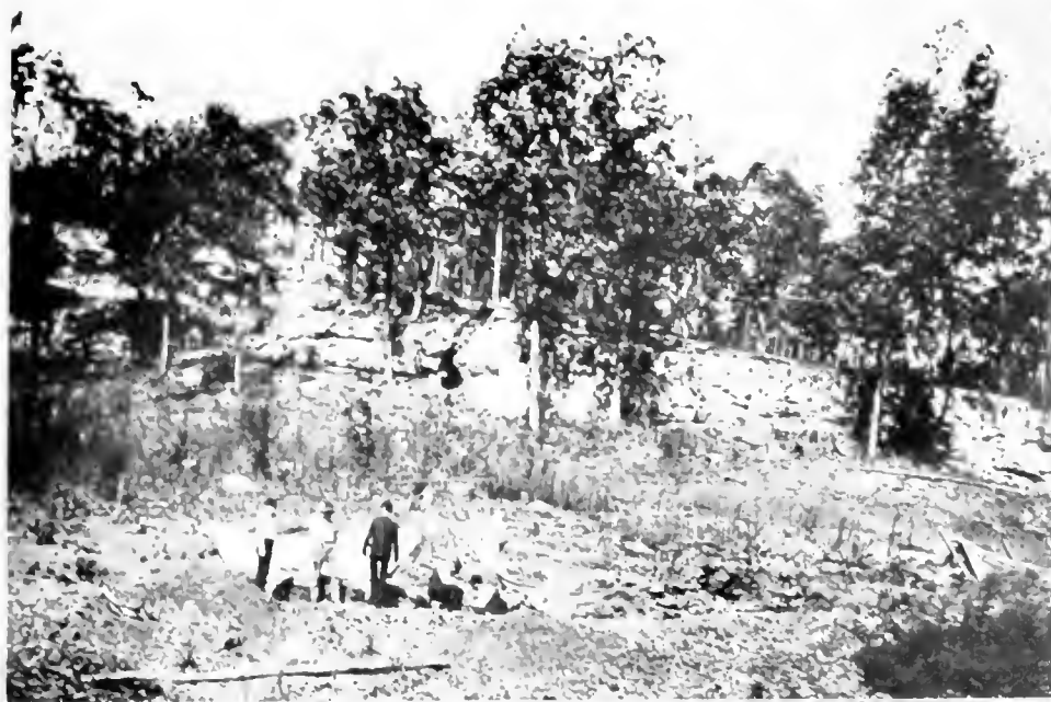
EXCAVATING FOR VASTOGEN SKELETONS IN SUBURBS OF ST. LOUIS
