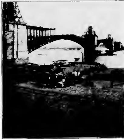
EADS BRIDGE NEARING COMPLETION
