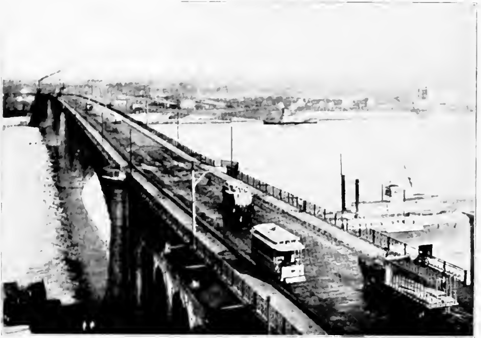
UPPER ROADWAY OF THE EADS BRIDGE
