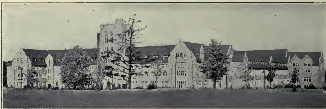
Loretto Abbey (of the Holy Family), founded 1847. Armour Heights, Toronto. Mother House and Novitiate of the I.B.V.M. in America. School for resident and non-resident pupils. Complete course from Kindergarten to Honour Matriculation, University of Toronto. Music, Art, Commercial Subjects. Athletics, etc. Convents, 15. Separate and Parochial Schools, 29.
