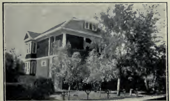
Loretto Convent (of Regina Angelorum), 1932. Regina, Saskatchewan. Residence for Sisters in Parochial School. Social Service, Sodality, etc.
