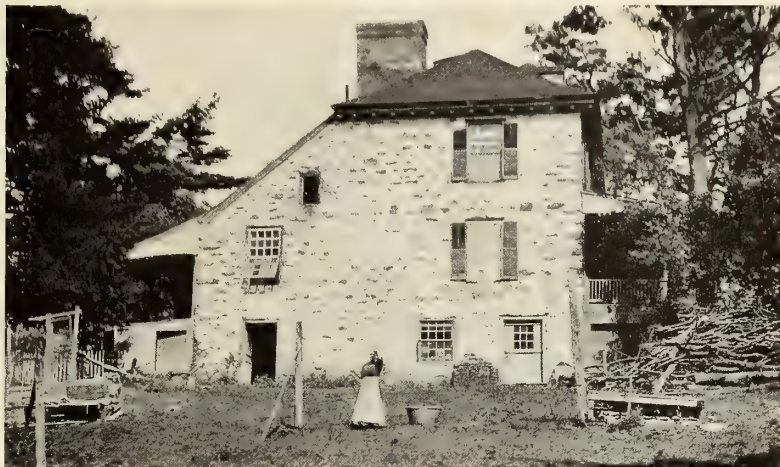
THE WEST END, SHOWING THE SOLID STONEMWORK.
