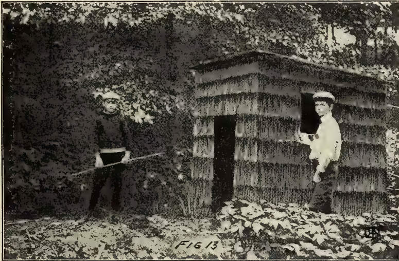
BUILDING A BRUSH CAMP
