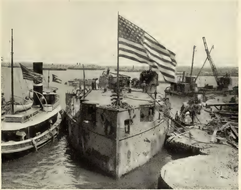
THE AFTER PORTION OF THE "MAINE" FLOATED OUT OF THE COFFER-DAM AND READY TO BE BURIED AT SEA WITH HONORS.
