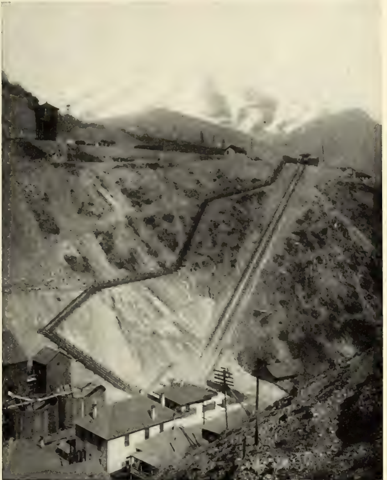
THE INCLINED RAILWAY FROM THE TOWN OF BINGHAM UP TO THE HIGH LINE RAILROAD. Six hundred feet difference in the levels.
