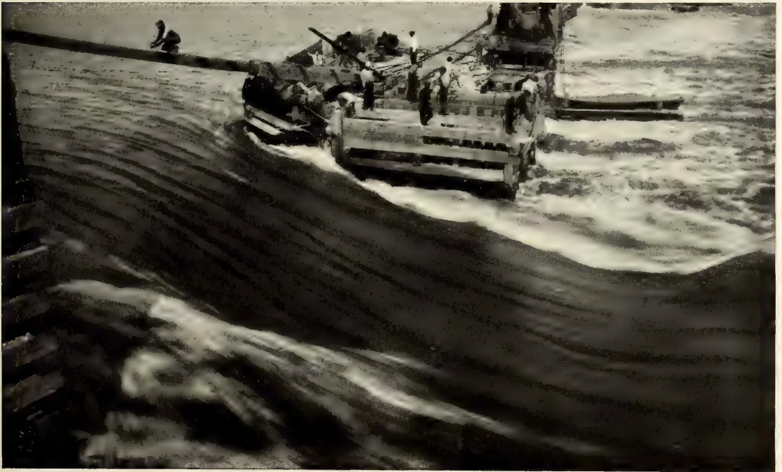
THE FINAL STRUGGLE OF THE RIVER AS THE LAST GAP WAS BEING CLOSED.
