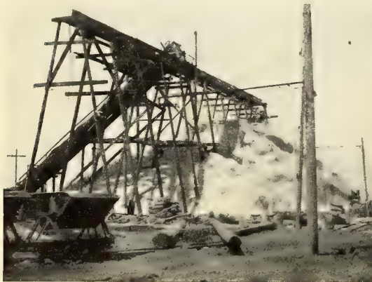
A PILE OF SALT UNDER THE WASHER AND STACKER, READY FOR SHIPMENT.
