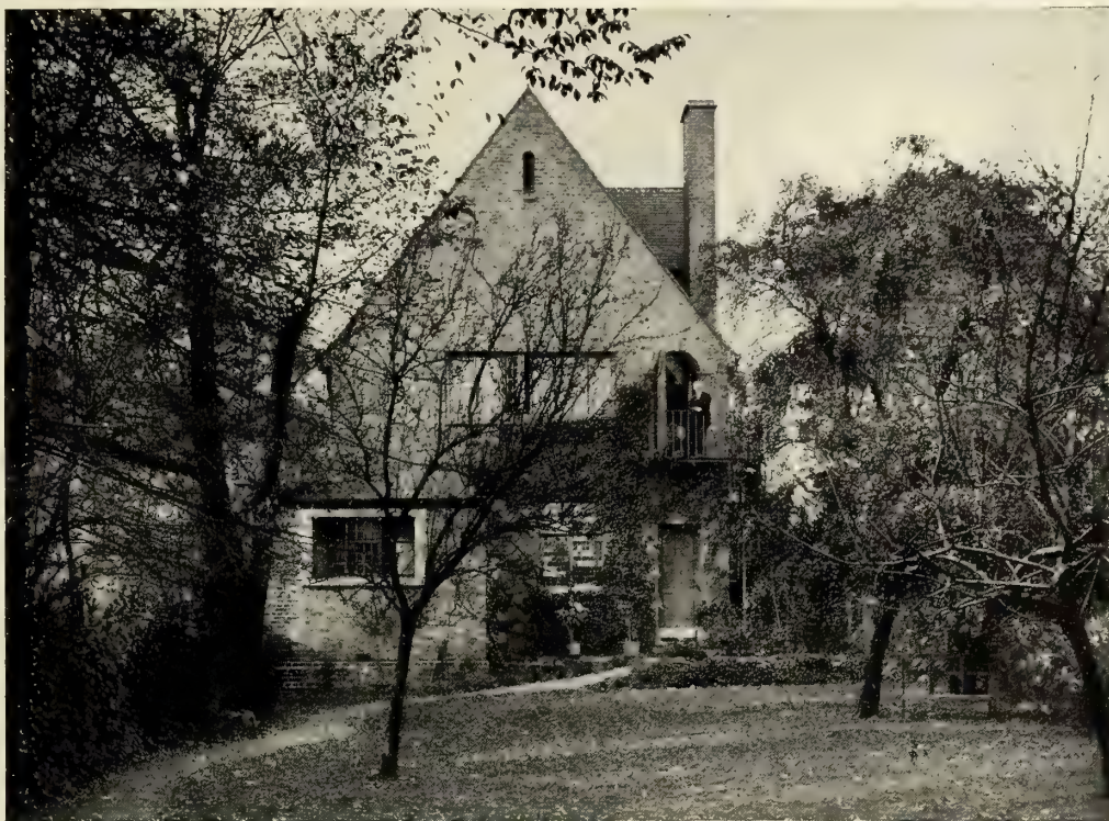
MR. RACKHAM'S HOUSE IN CHALCOT GARDENS, SOUTH HAMPSTEAD, LONDON.
