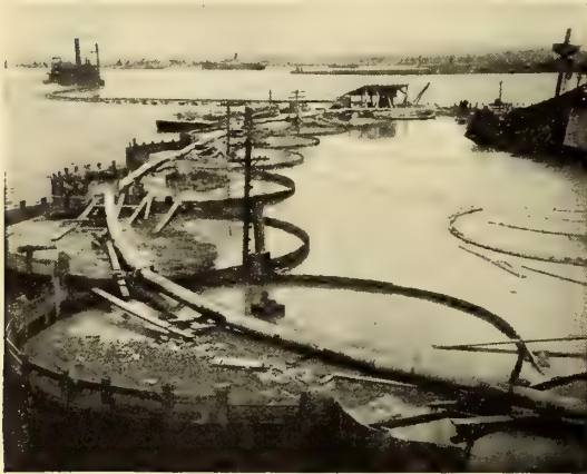
THE DREDGE (IN THE DISTANCE) PUMPING THE CYLINDERS FULL OF CLAY.
