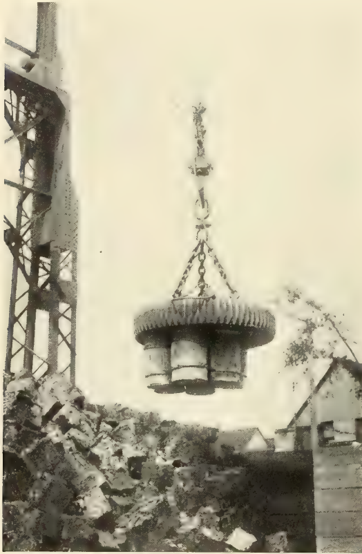
SEVEN KEGS FILLED WITH NAILS LIFTED BY AN ELECTRO-MAGNET.
