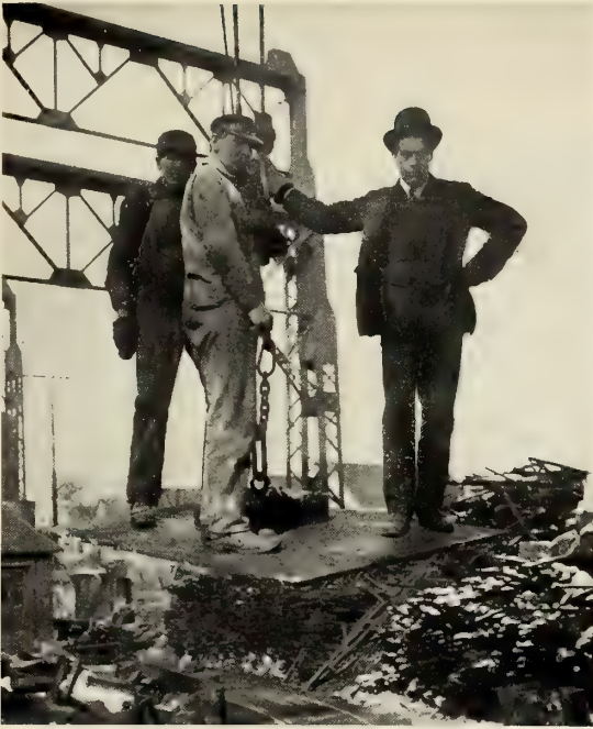
STANDING ON A SHEET OF STEEL WHICH IS GRIPPED AND HELD BY THE UNSEEN POWER OF THE MAGNET.
