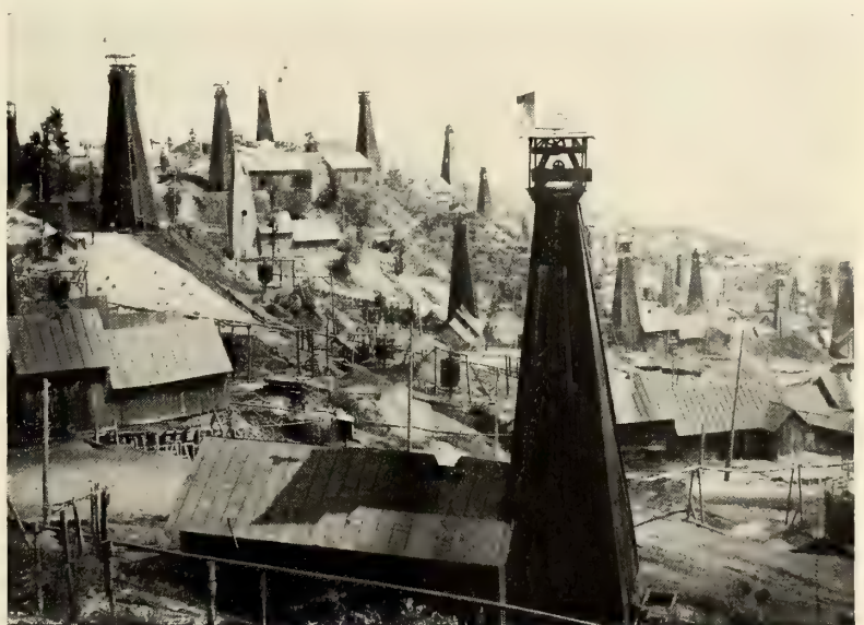
THE CURIOUS RUMANIAN OIL-DERRICKS.
