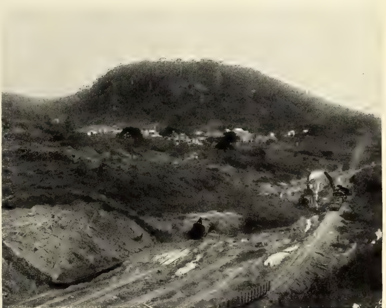
THE CUCARACHA SLIDE MAKING MORE WORK FOR THE CANAL DIGGERS.
