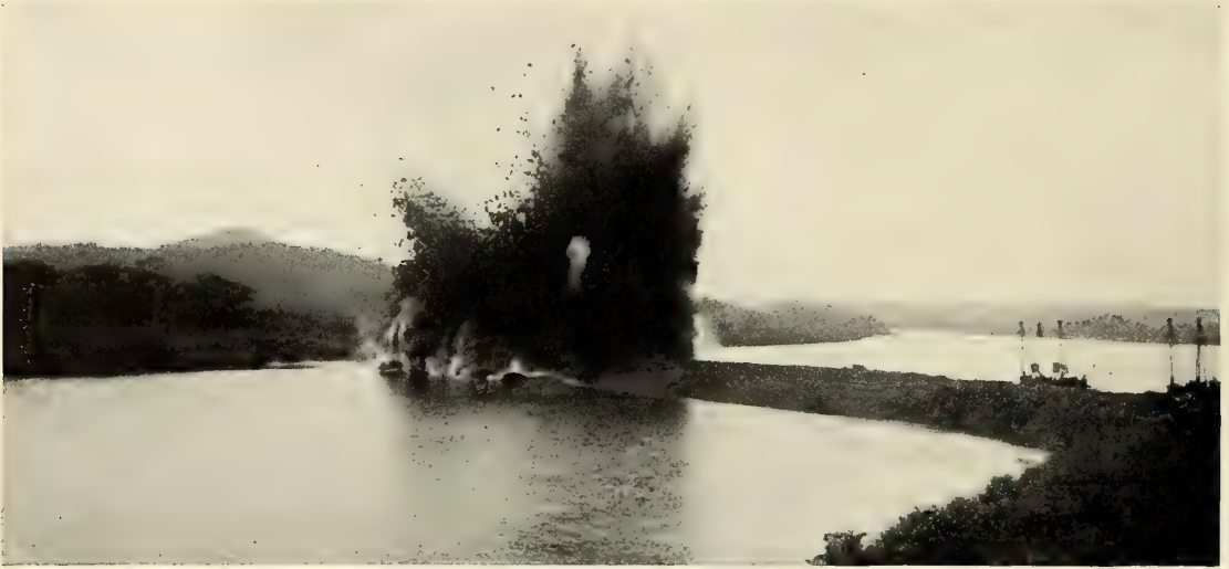
THE ISTHMUS SEVERED! FORTY TONS OF DYNAMITE SHATTERING THE GAMBOA DIKE.
