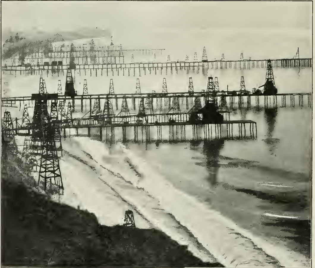
DERRICKS FOR PUMPING OIL FROM THE OIL-SAND FAR BELOW THE WATER NEAR SANTA BARBARA.
