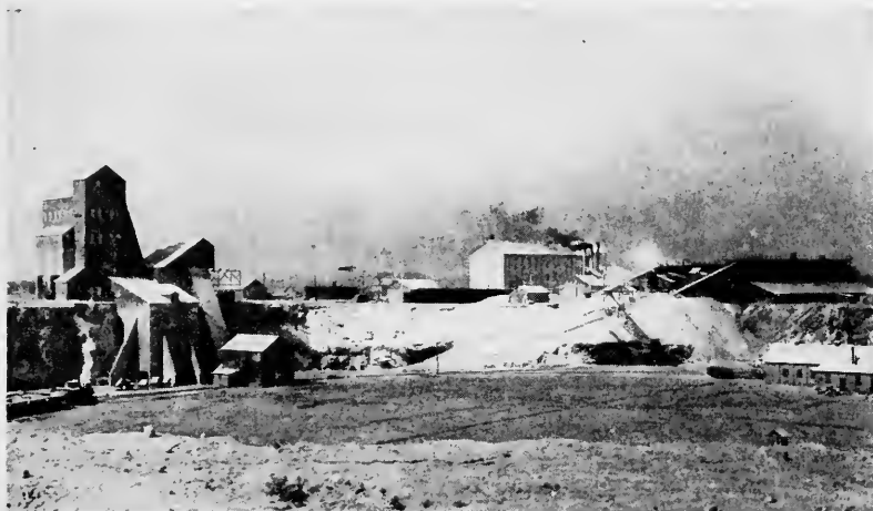
FIG. 68.—A typical Ohio lime plant and quarry with supplementary crushing and screening plant shown at left.
