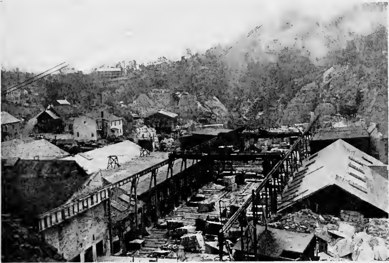
FIG. 58.—Two soapstone saw mills with overhead traveling crane between them, Schuyler, Va. (Photo by H. Herbert Hughes.)
