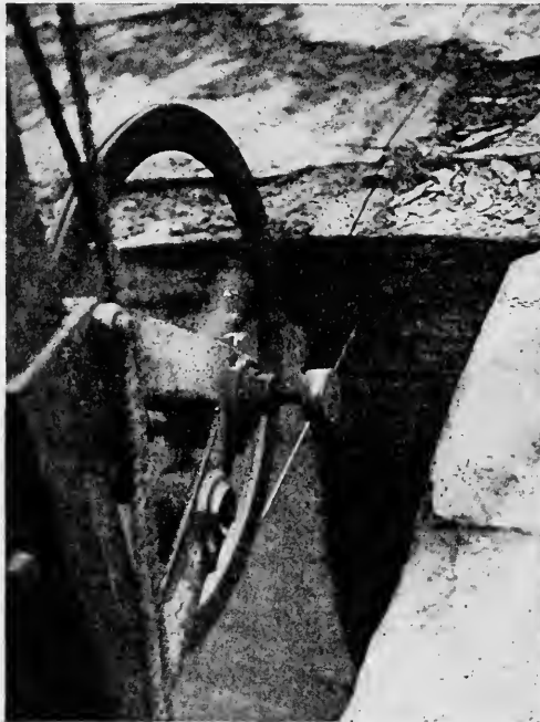
FIG. 46.—Wire saw at the point where it leaves the cut.
