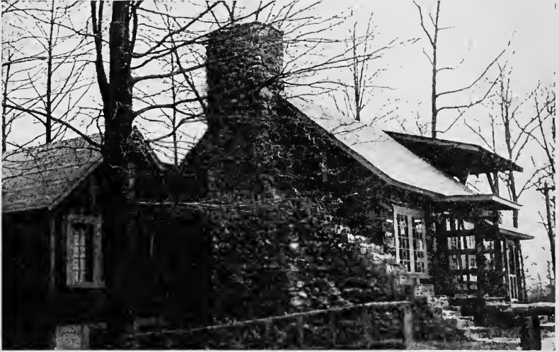
FIG. 60.—A unique type of boulder construction combining chimney with stairway. (Photo by H. Herbert Hughes.)
