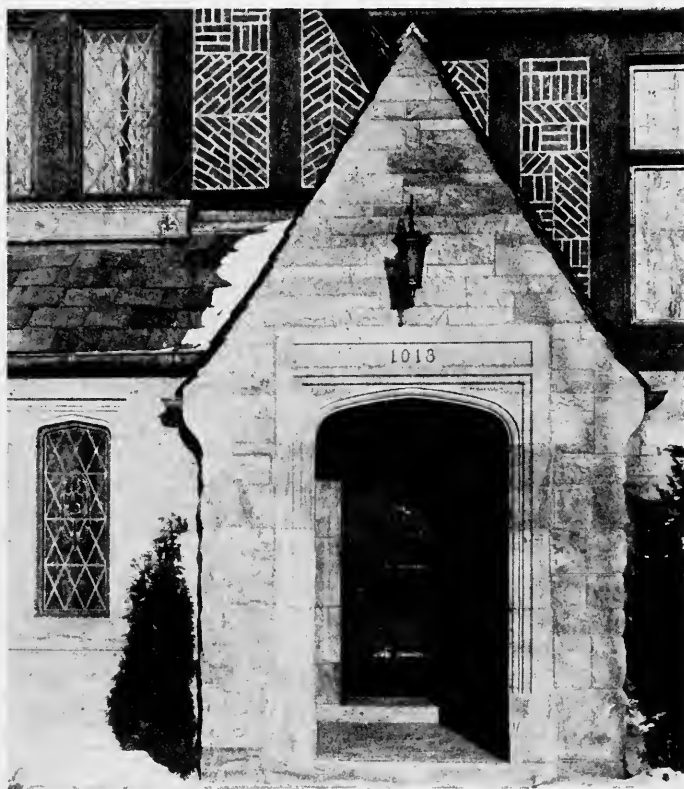
FIG. 13.—An attractive use of sandstone ashlar. (Courtesy of Briar Hill Stone Company.)
