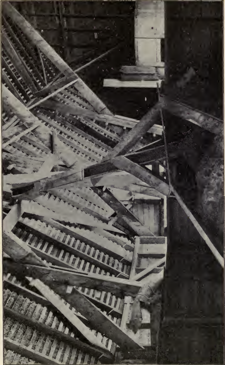
PLATE VIII. ELEVATORS AND BINS ON SECOND FLOOR.
