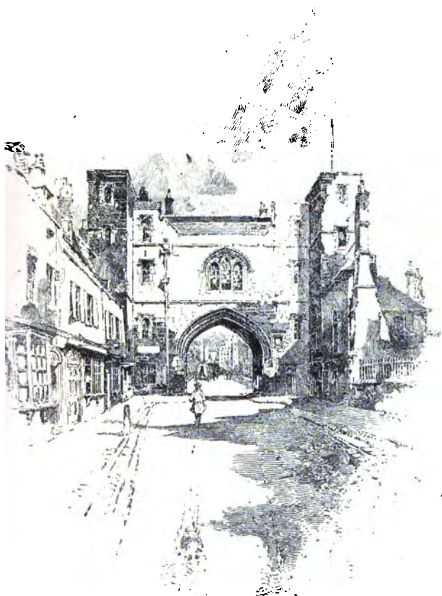
St John's Gate Ipswich Residence of Edward Cole 1851
