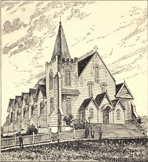
THE METLAKAHTLA CHURCH : BUILT ENTIRELY BY THE NATIVES.
