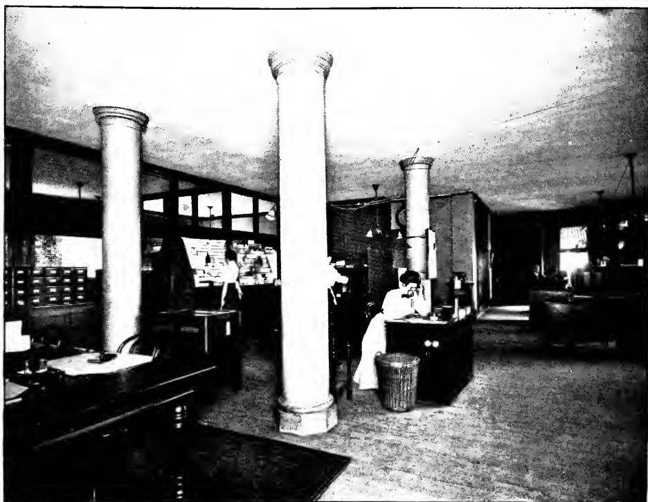
THE "ROOMS" IN 1860 AND 1910 THE BOARD'S BUILDING IN PEMBERTON SQUARE THE GENERAL OFFICE IN THE CONGREGATIONAL HOUSE
