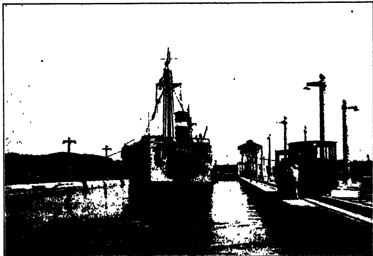
PANAMA CANAL: at the Miraflores Locks, looking north, showing S. S. Santa Clara in lower west chamber, ready for water to be lowered to sea level.
