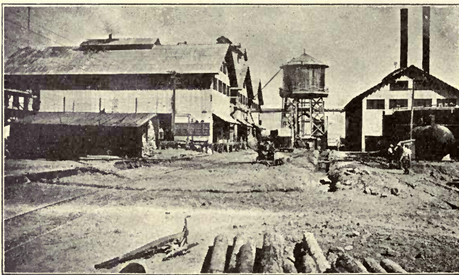
The plants shown in Fig. 22 are the Borosolvay plants of the Pacific Coast Borax Company and the Solvay Process Company at Searles Lake, California. All of this region is rich in borax and potash deposits, and electricity is used extensively in the recovery process. Over 11,000,000 kw-hr. were used by the chemical plants of this vicinity in 1920.
