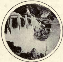
25 HP IN THE POWER PLANT
