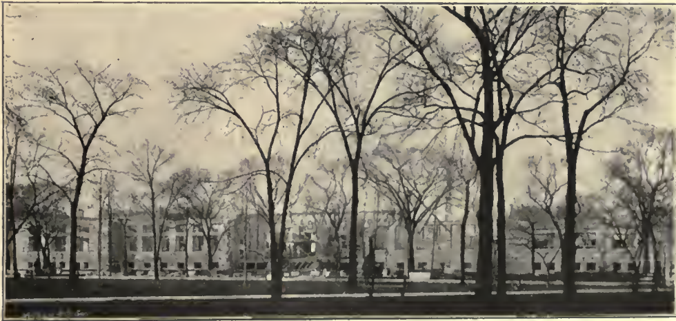
NEWBERRY LIBRARY BUILDING, (Under construction January 1st, 1892.)
