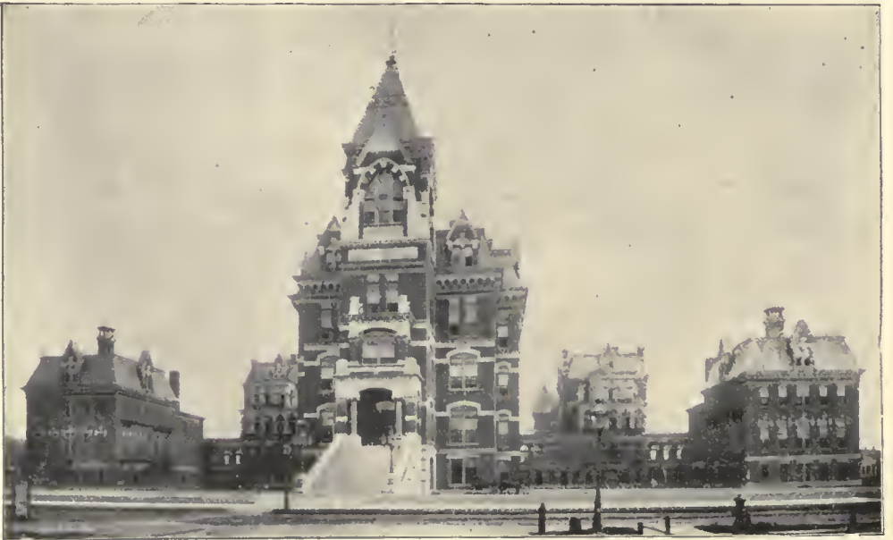
COOK COUNTY HOSPITAL, HARRISON STREET.
