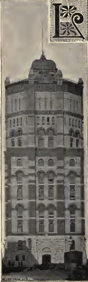
PULLMAN WATER TOWER.
