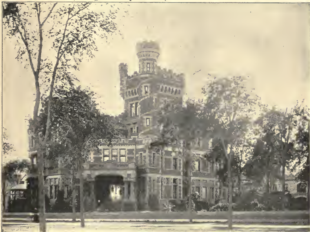
POTTER PALMER'S RESIDENCE ON LAKE-SHORE DRIVE.
