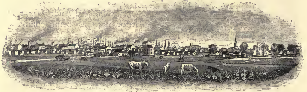
CHICAGO IN 1845, FROM THE WEST.
