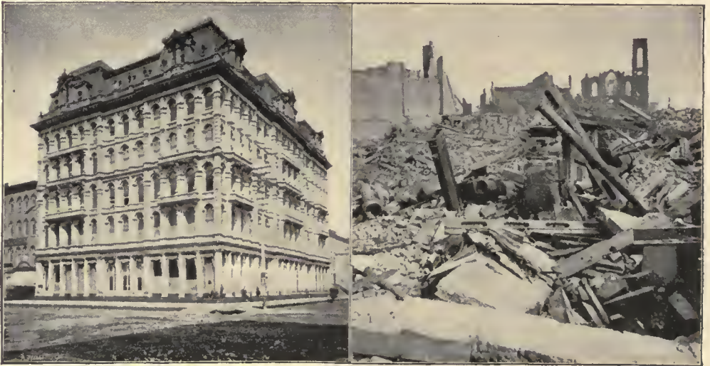
FIELD & LEITER'S STORE, BEFORE AND AFTER THE FIRE OF 1871.
