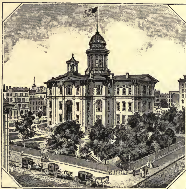
THE SECOND COURT-HOUSE, WITH ITS ADDED STORY.
