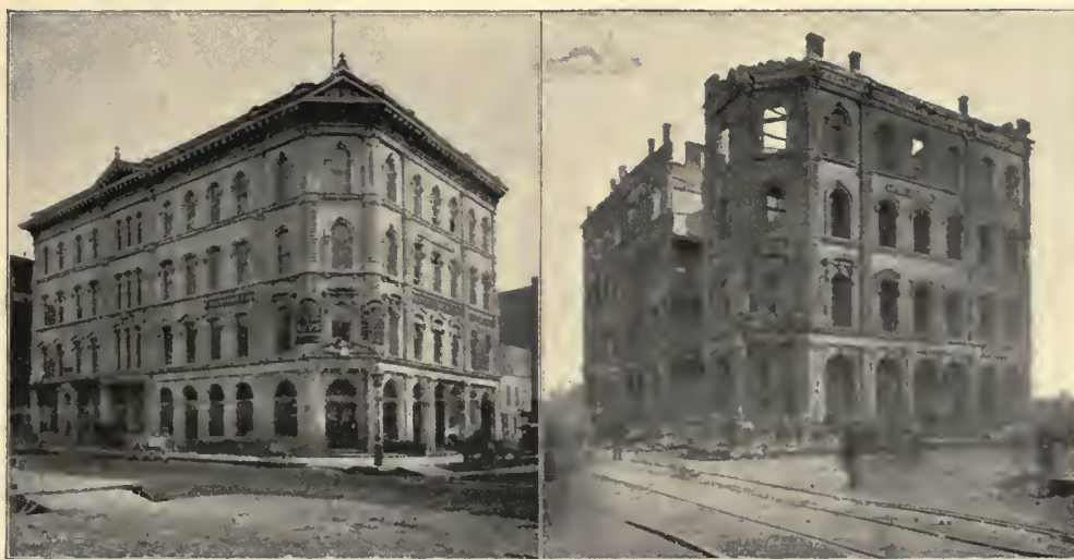
TRIBUNE BUILDING, BEFORE AND AFTER THE FIRE OF 1871.
