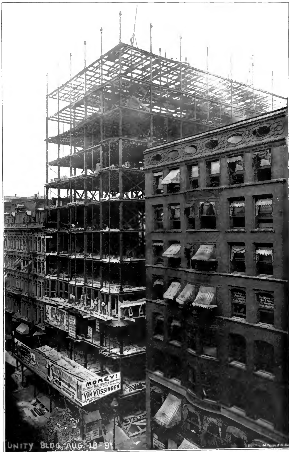
"THE CHICAGO CONSTRUCTION," A FRAME THAT HOLDS UP THE WALLS.
