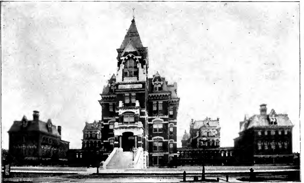
COOK COUNTY HOSPITAL, HARRISON STREET.
