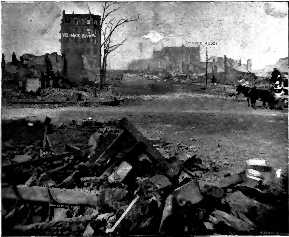
WASHINGTON STREET, WEST FROM WABASH AVENUE, OCTOBER 17, 1871.
