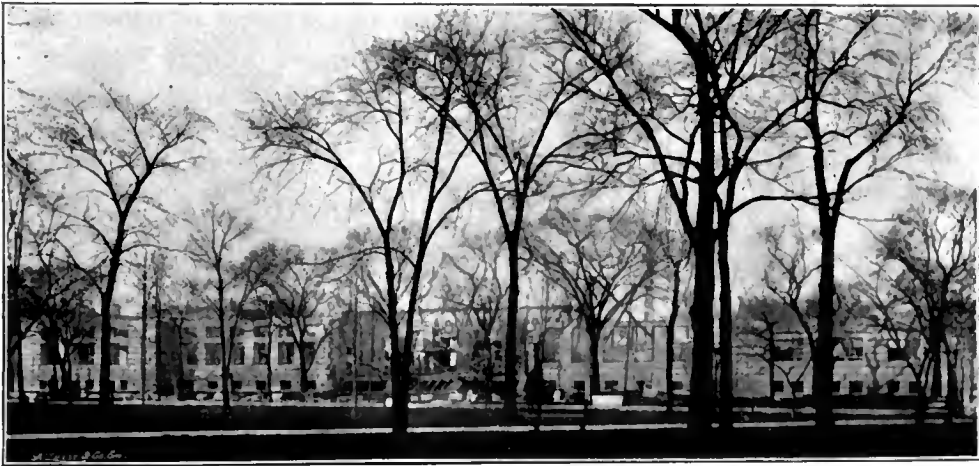
NEWBERRY LIBRARY BUILDING, (Under construction January 1st, 1892.)
