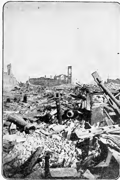
RUINS OF FIELD & LEITER BUILDING.
