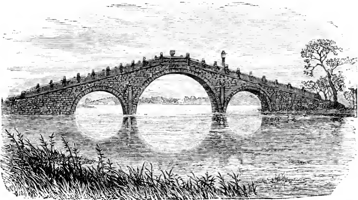
BRIDGE IN CHEH-KIANG.
