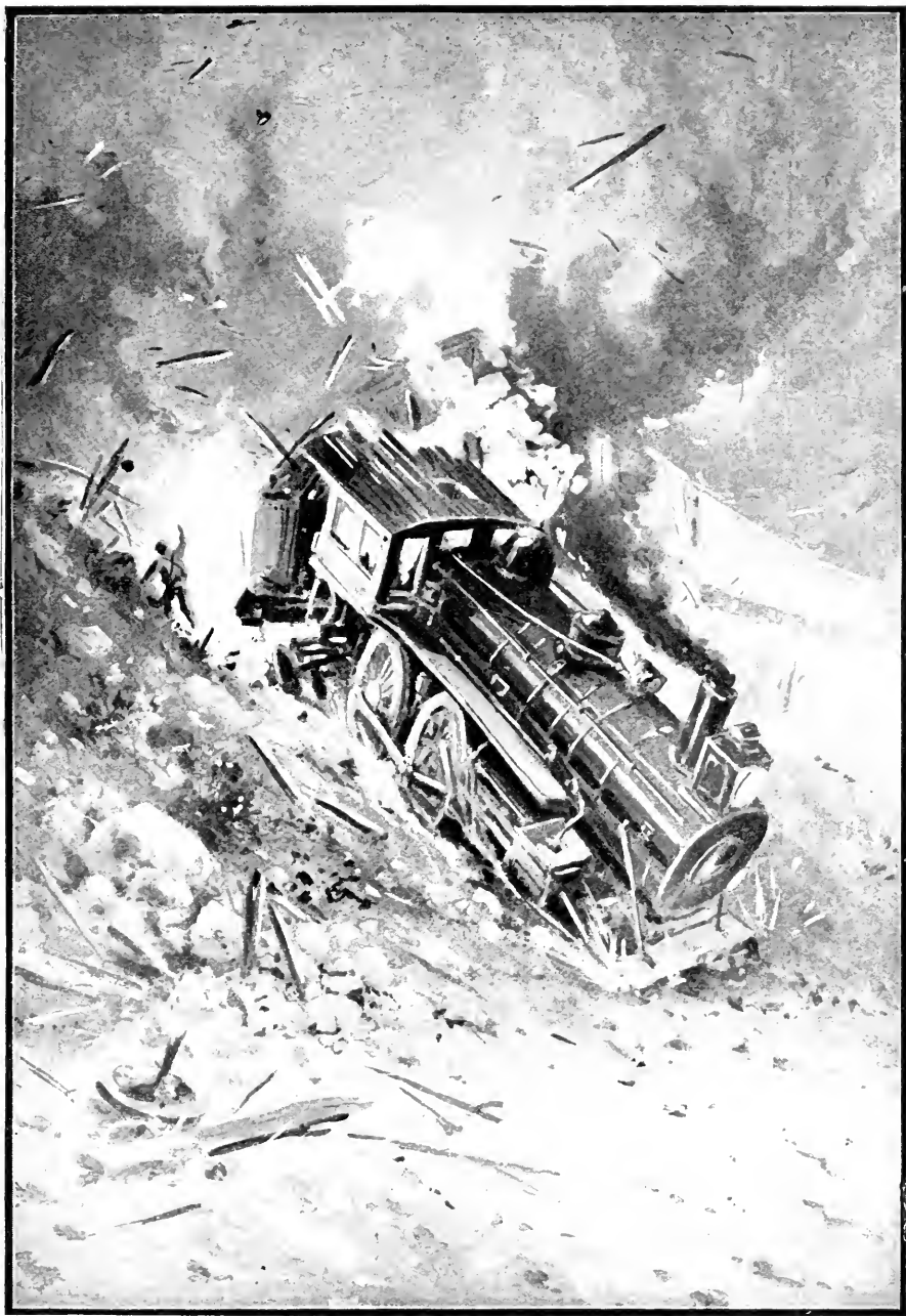
DESTRUCTION OF RAILROAD TRAIN BY DYNAMITE
