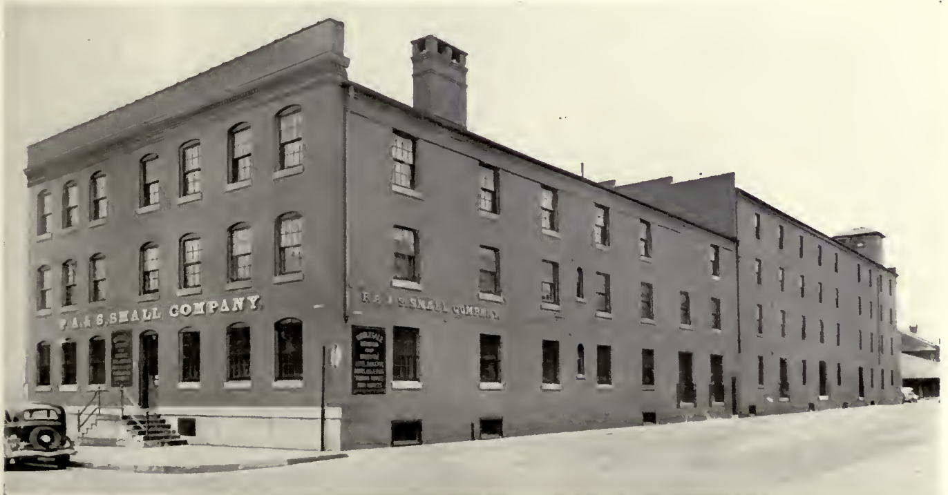
Hardware and Grocery Warehouse.
