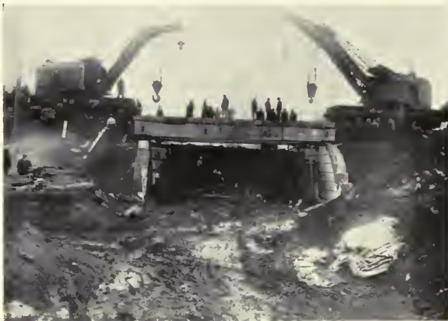
W.M.R.R. Overpass, Franklin County
