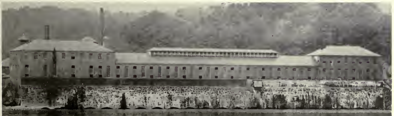
Hydroelectric Station on Susquehanna River at York Haven
