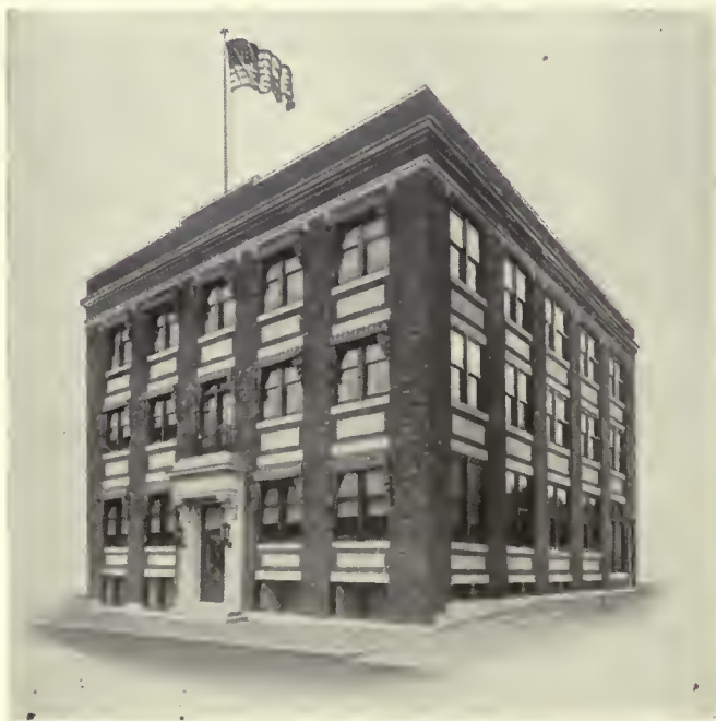
The building of the Manufacturers' Association.
