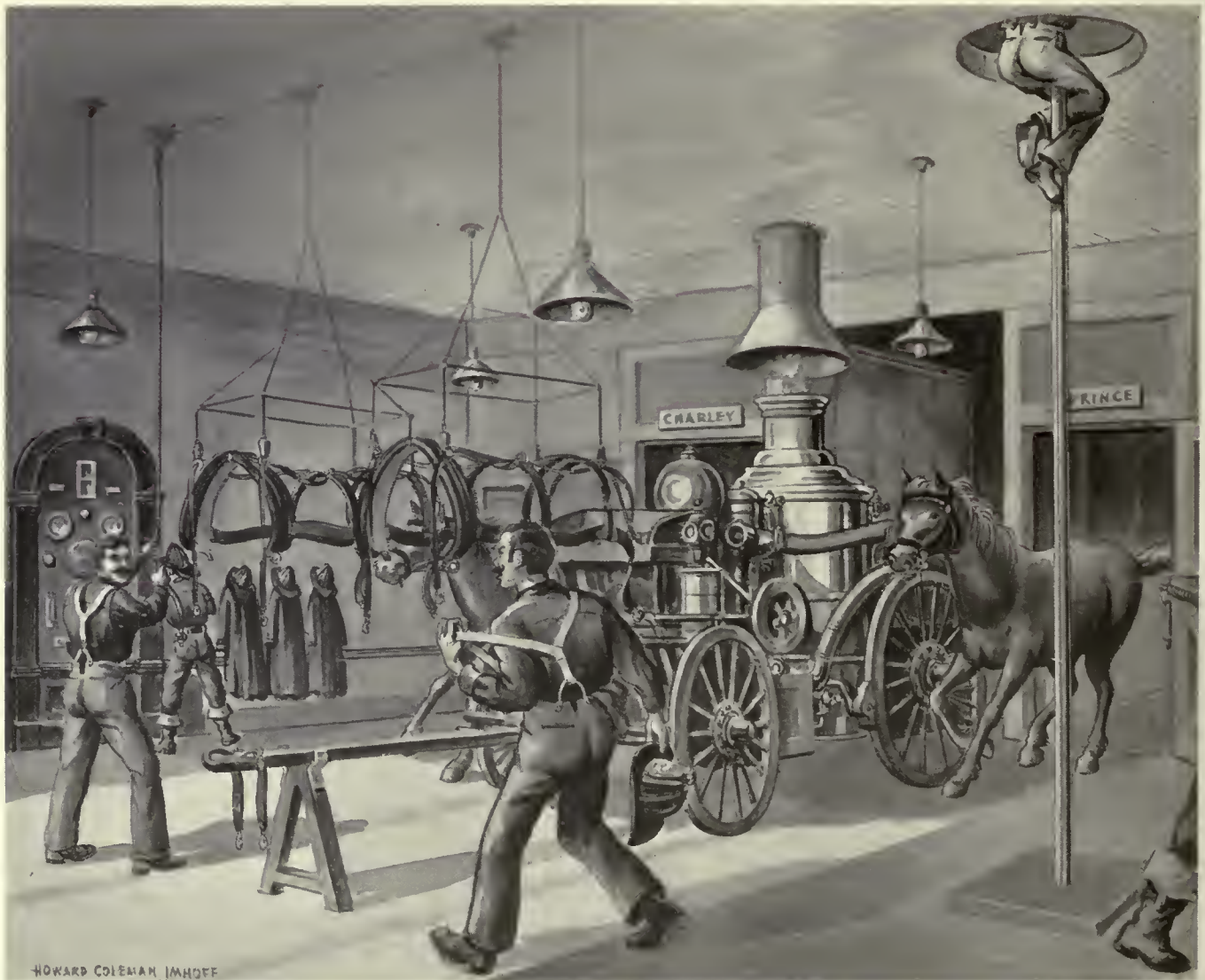
The romance of the horse-drawn steam fire engine. When the alarm went off, the stall doors slid open and the horses dashed to their places in front of the fire engine. The harness dropped down upon their backs, and they were off in a cloud of dust.
