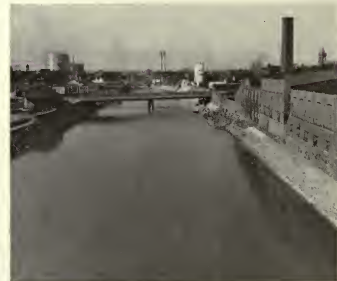
The channel deepened, widened and faced with stone.
