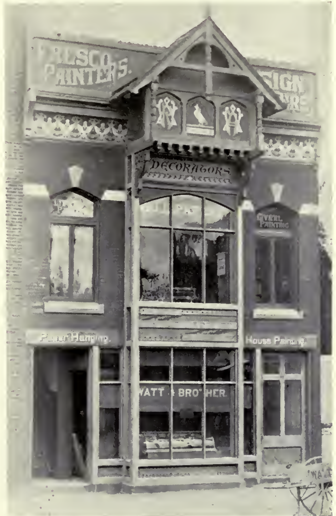
Old Laurel Fire House, Home of Watt & Brother in 1878.
