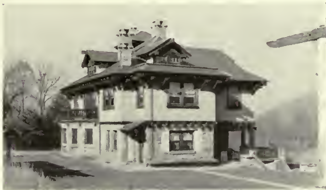
Indian Steps Museum, built by J. Edward Vandersloot.
