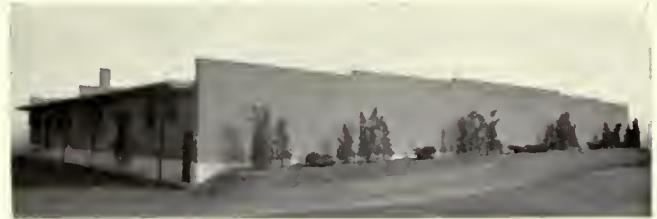
General Storage Warehouse.
