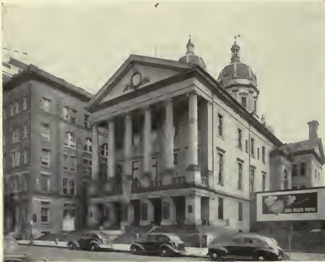
York County Courthouse and Annex.
