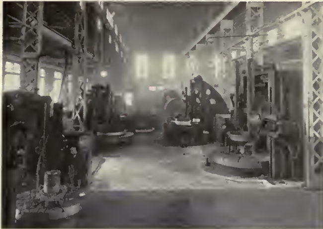
Large Vertical Boring Mill Section of Machine Shop.
