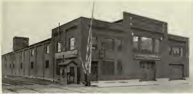
Pipe and Steel Warehouse.
