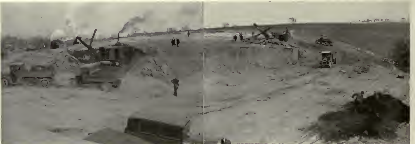
Excavation, York Hospital, York, Pa.
