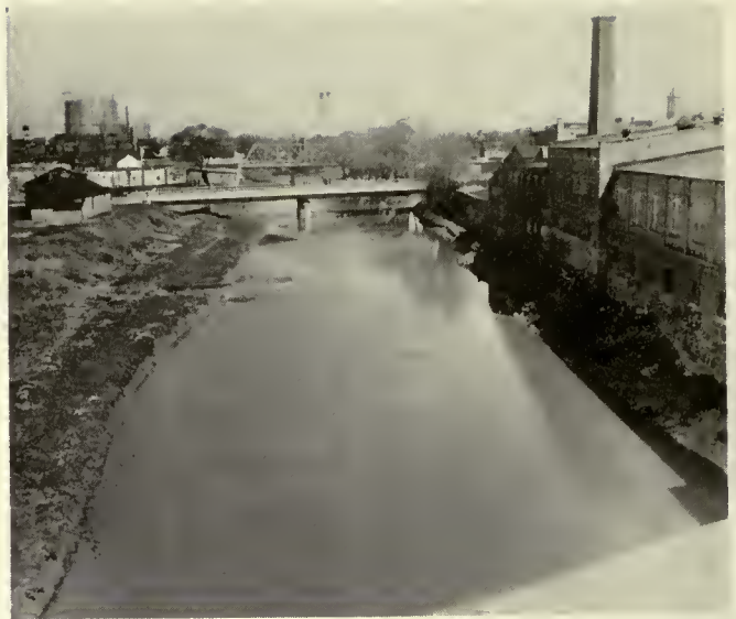
The Codorus before Flood Control, Princess Street Bridge.
