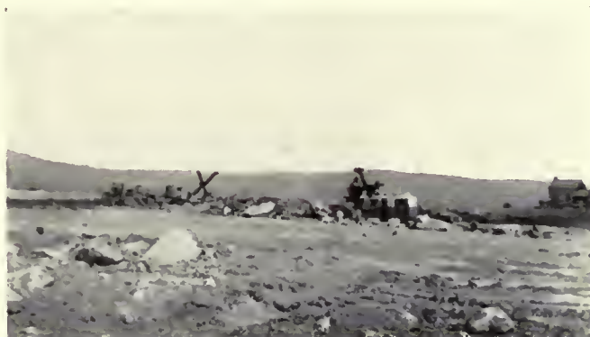
Airport Excavation, Allentown, Pa.
