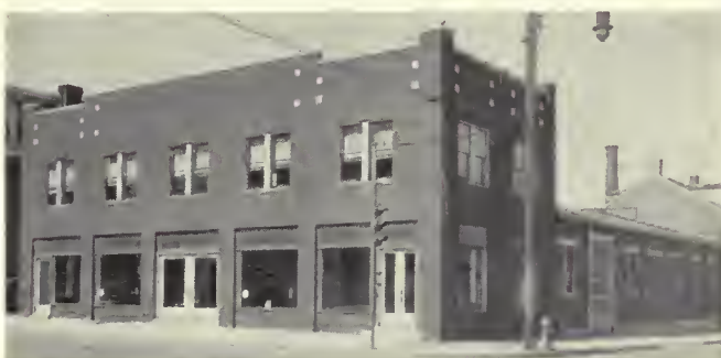
General Office, Showroom and Service Department.
