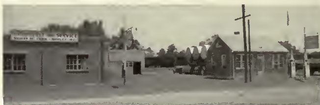
Bulk Plant, Storage and Office.
