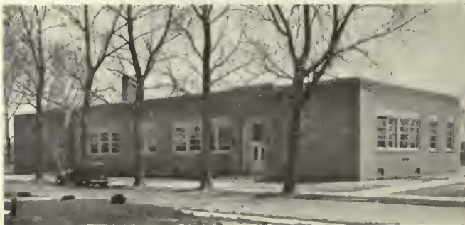
Franklin Elementary School Annex.
