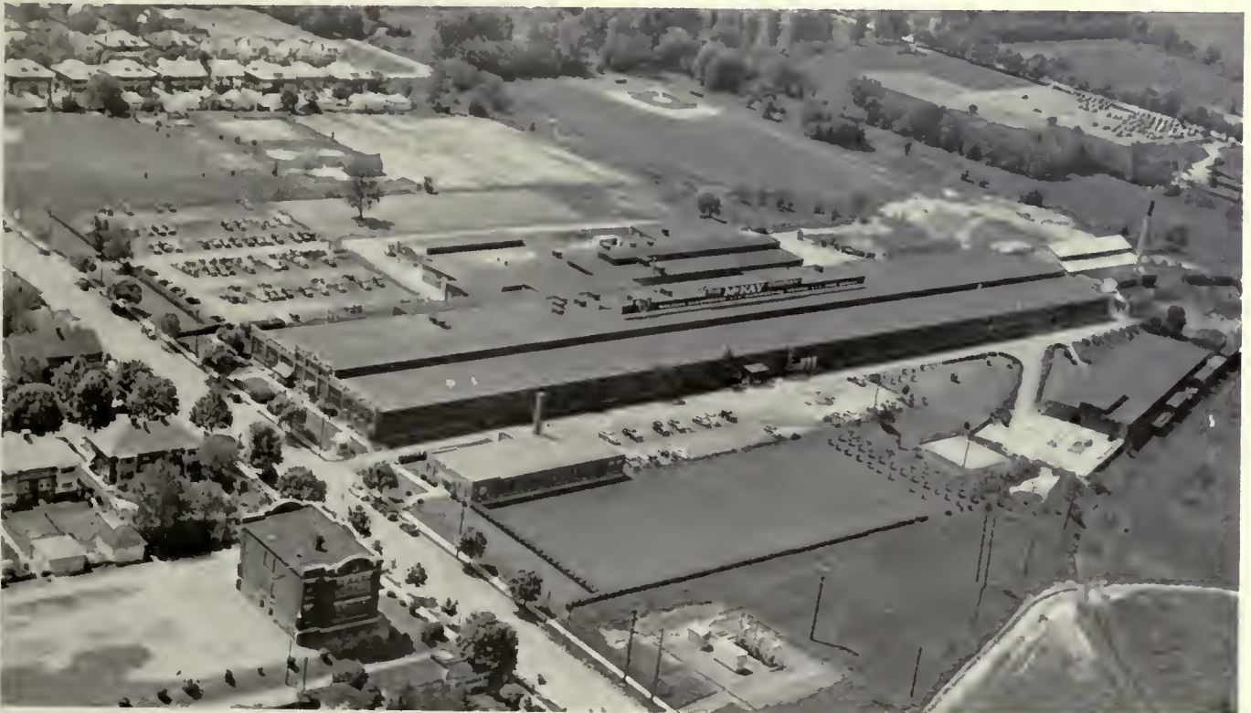
Aerial View of York Plant.
