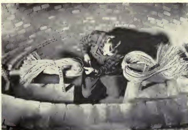
Connecting Underground Telephone Cables
