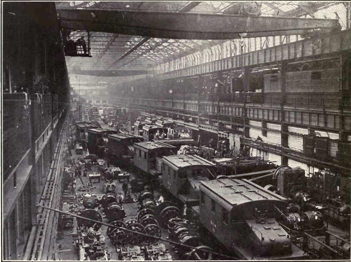
Equipping Electric Locomotives in the Westinghouse Works
