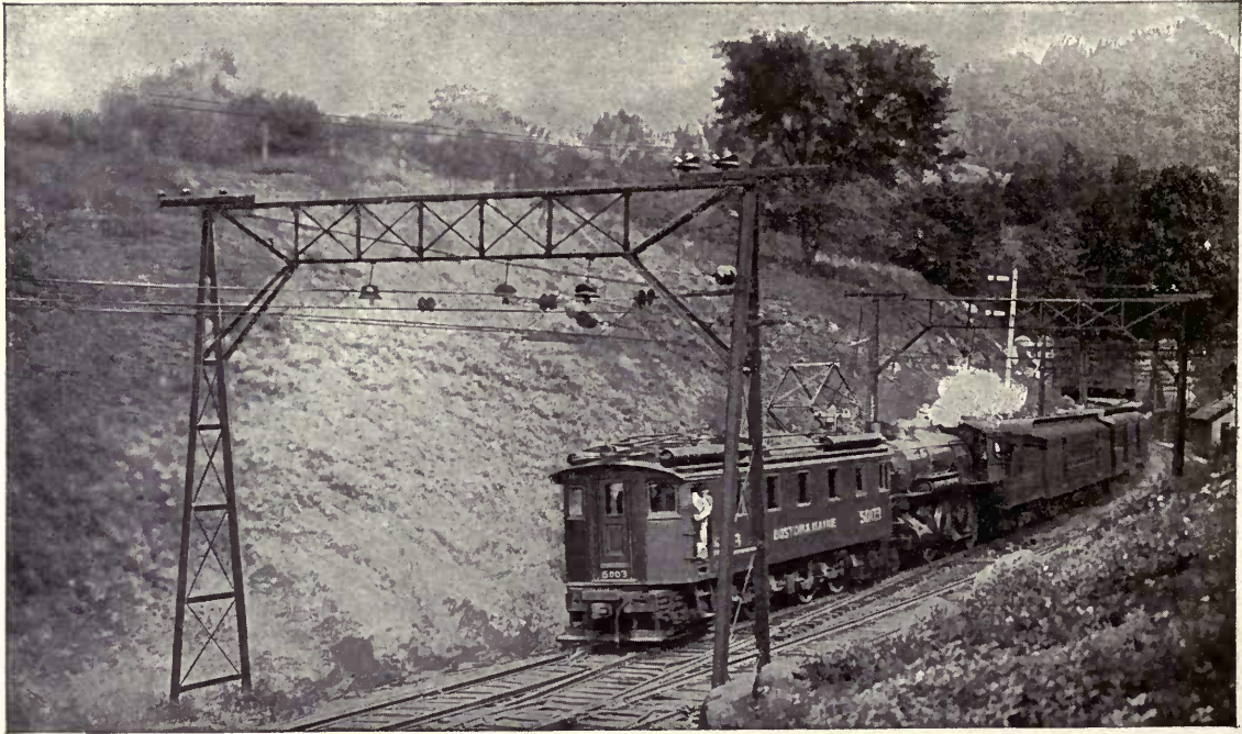
Typical Passenger Train in Electric Operation at Hoosac Tunnel. The Steam Locomotives Are Hauled Through with Banked Fires. Three Trains in Each Direction Are Now Allowed in the Tunnel
