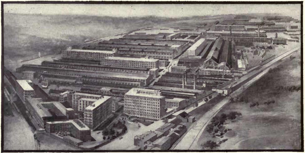
General View of the Schenectady Works, General Electric Company
