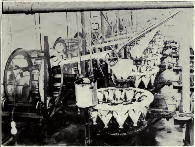
Can-filling machines. These automatic machines are great labor-saving devices, filling the cans with fruit or vegetables direct from the cooker
