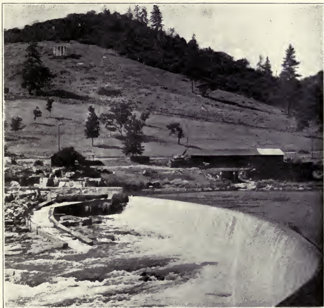
A "fish ladder" on Rogue River, Oregon. By means of such ladders, salmon on their way up the river to the spawning grounds are helped over falls and dams
