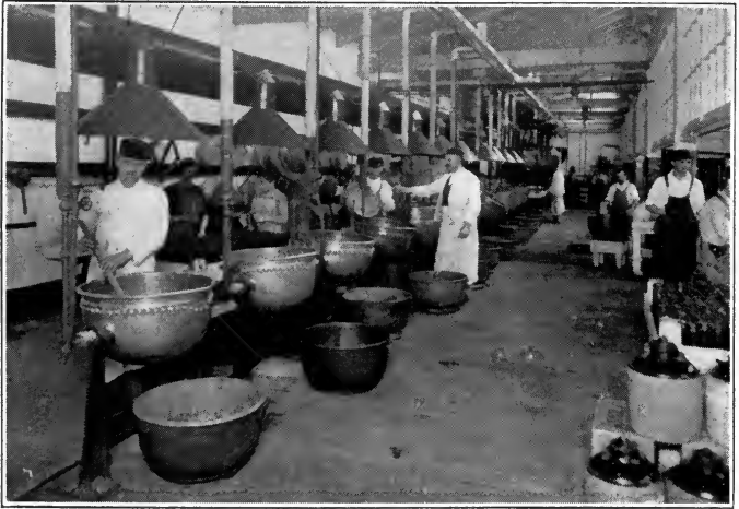
Transforming peaches into preserves in the great kettles or caldrons at the manufacturing plant of a wholesale food house
