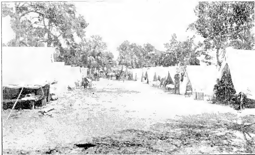
A COMPANY STREET.
