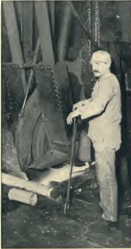
Cutting bars of steel in the Schneider works at Creusot, France. In organization and output these French munitions factories rival the famous Krupp works at Essen
