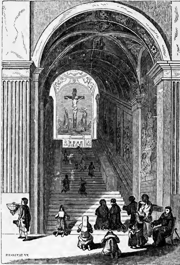
CLIMBING THE STAIRS.
