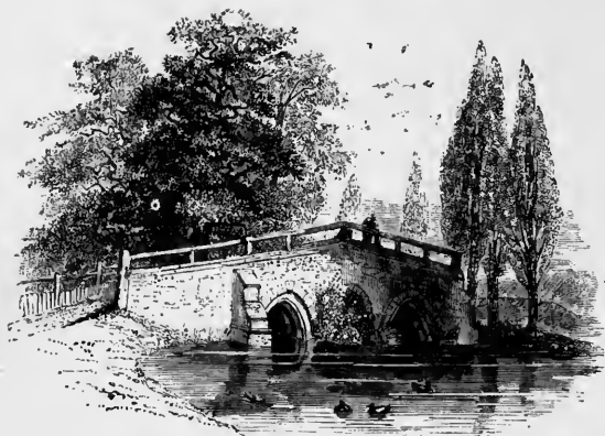
BRIDGE AT HADLEIGH.
