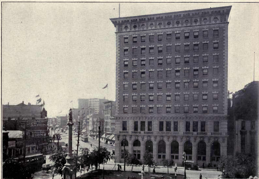
MAIN STREET, WINNIPEG, LOOKING SOUTH FROM THE CITY HALL
