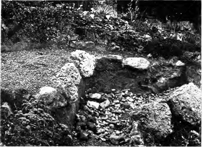
THE MORAINE IN COURSE OF CONSTRUCTION.
