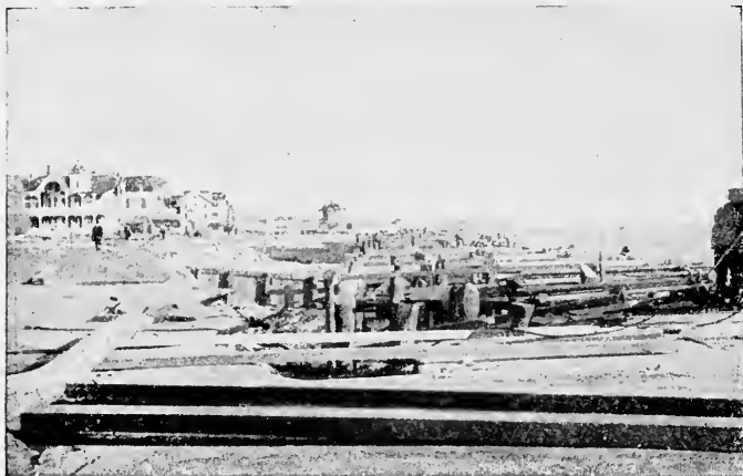
THE SEA CARRIED AWAY A PORTION OF THE WALK
