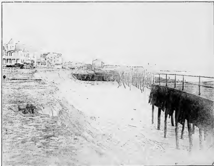
MANY OF THE PILING BARELY TOUCHING THE SAND
