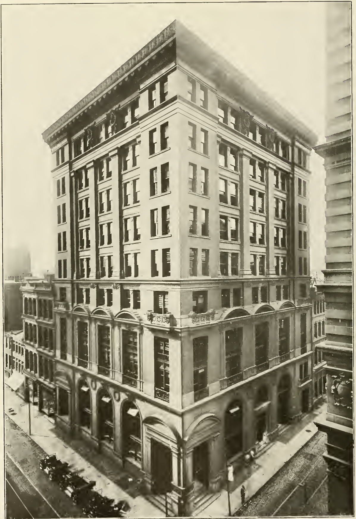
COLUMBIA NATIONAL BANK BUILDING
