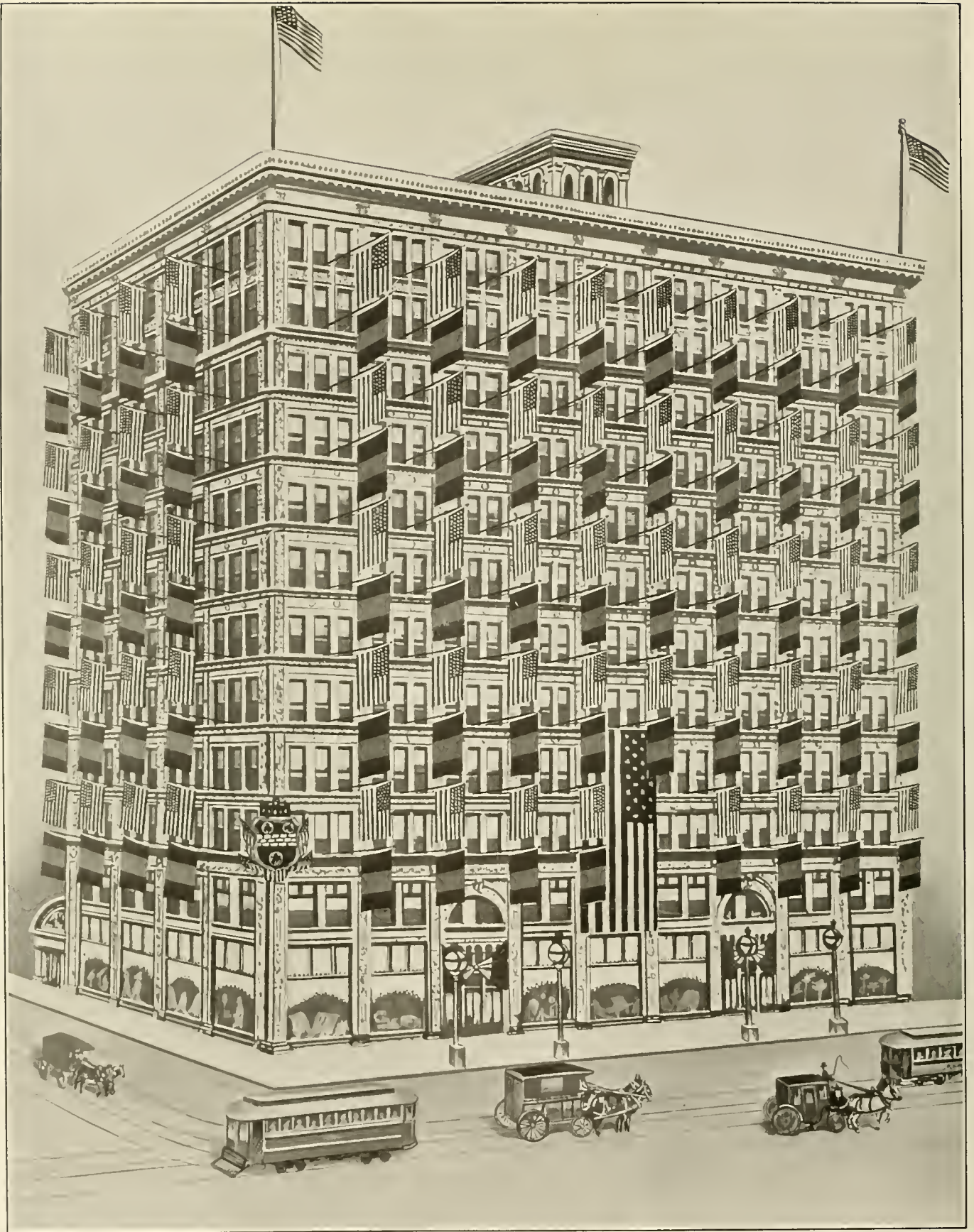
McCREERY BUILDING Finest decorated building in the city during the Sesqui-Centennial
