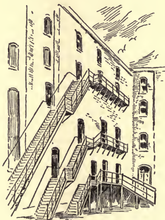
WEST FIRE ESCAPES.
