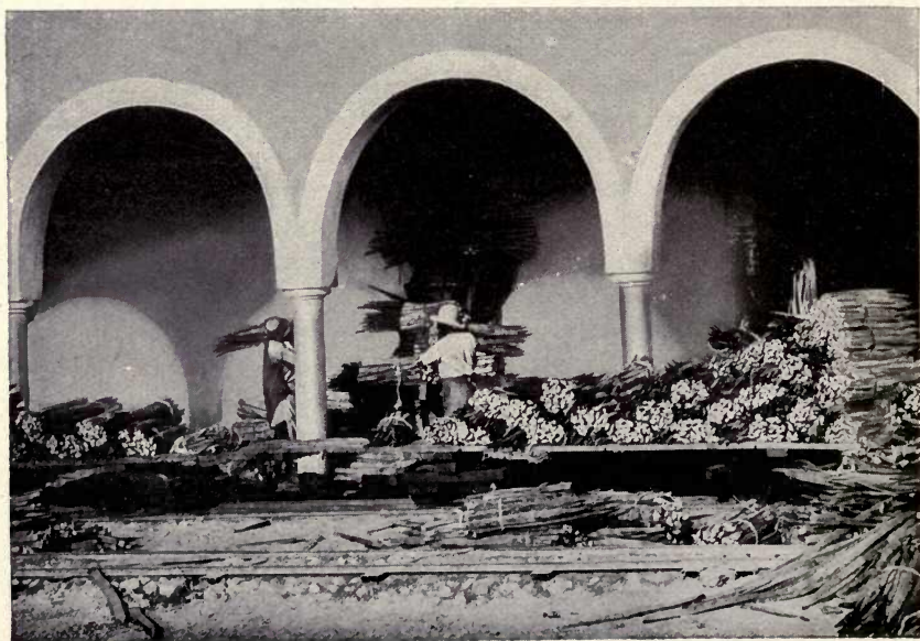
Exterior View of Decorticating Mill
