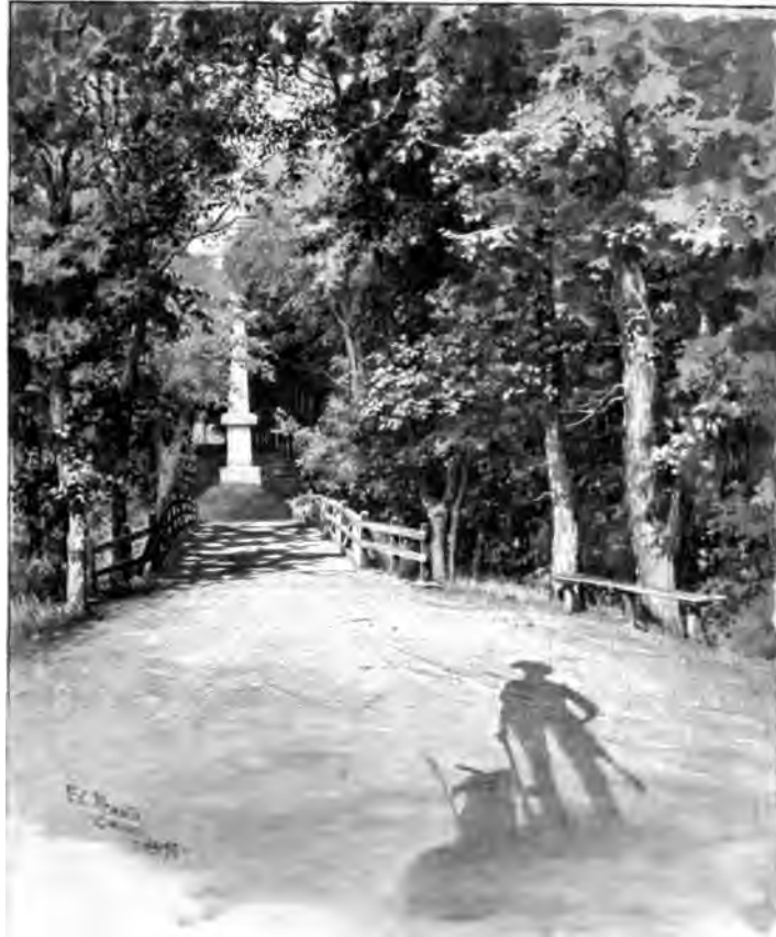
CONCORD BRIDGE AT THE PRESENT TIME.
