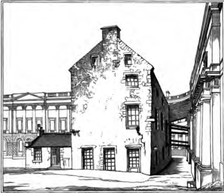
THE OLD LIBRARY (1823) FROM THE SOUTH.
