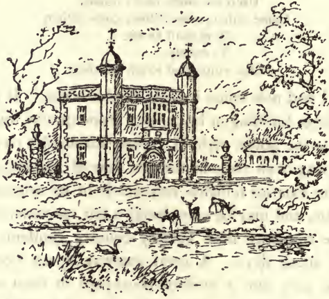
CHARLECOTE GATE HOUSE.
