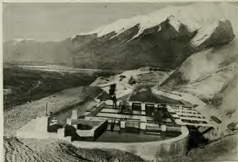
Forebay on Power Canal, Strawberry Valley Irrigation Project.
