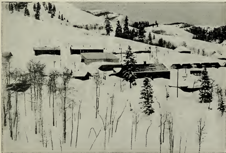
Water Shed, West Portal Strawberry Tunnel.
