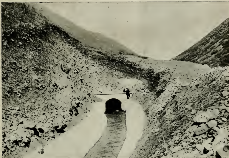
East Portal Power Plant Tunnel No. 1, Strawberry Project.
