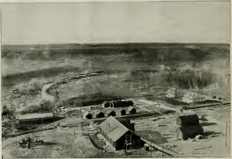
Power Plant, Strawberry Valley Irrigation Project.
