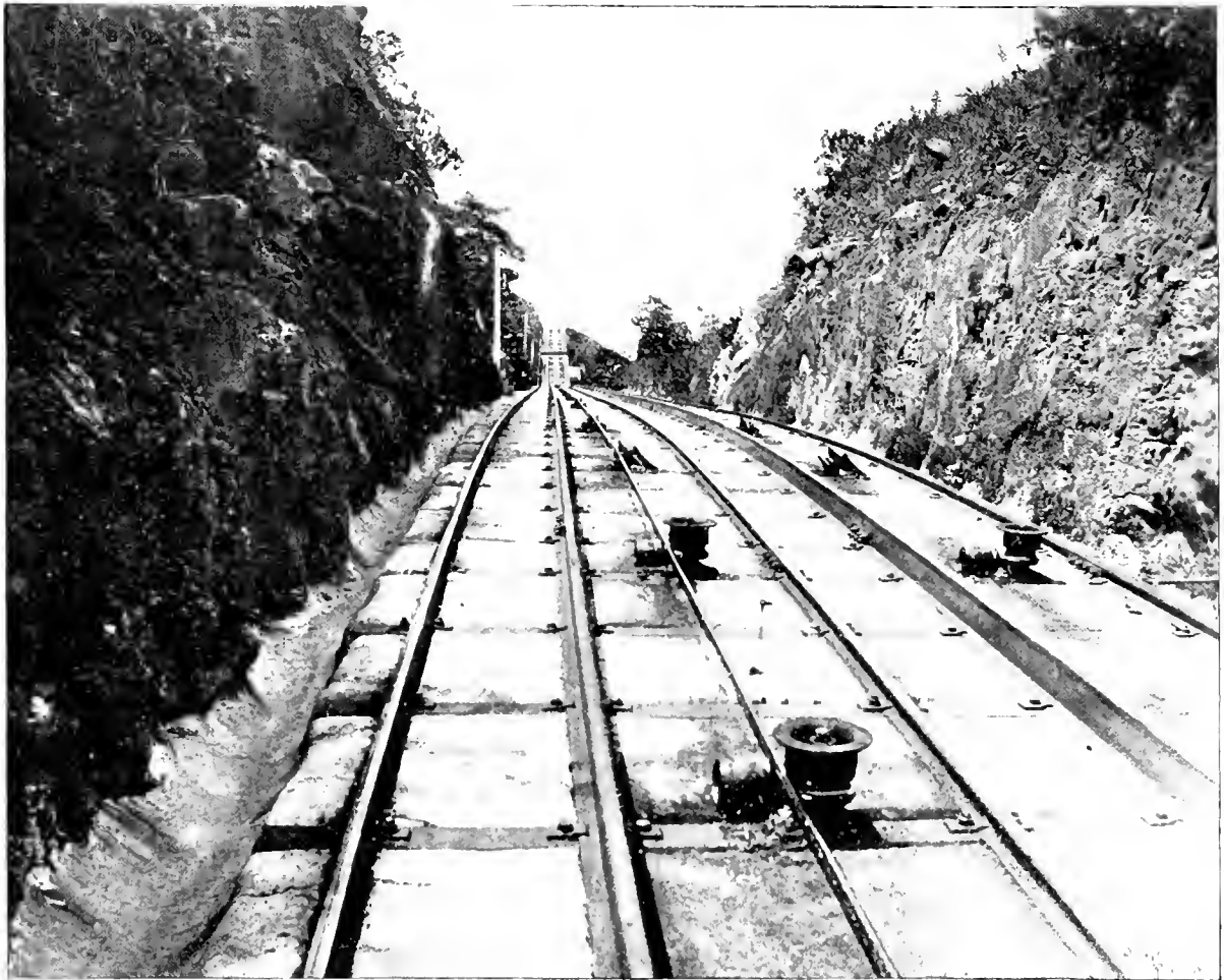
HONG KONG CABLE—ONE CAR ABOVE AND ONE CAR BELOW POINT WHERE PHOTOGRAPH IS TAKEN.
