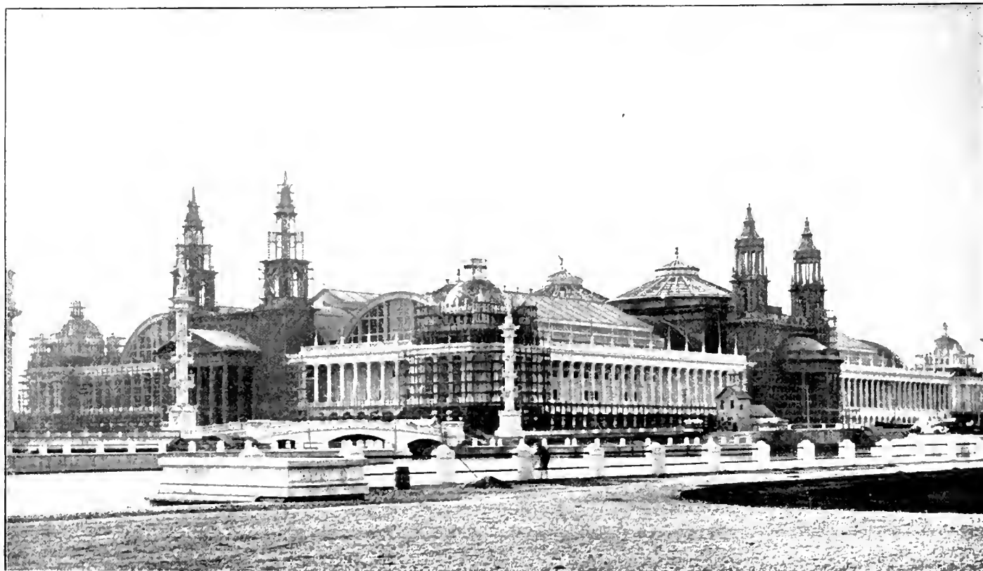
MACHINERY HALL — THE LAST IN EXTERIOR COMPLETION.
