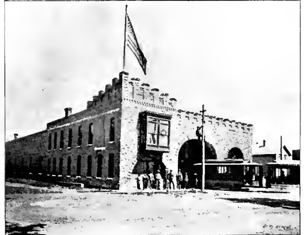
FRONT EXTERIOR VIEW.
