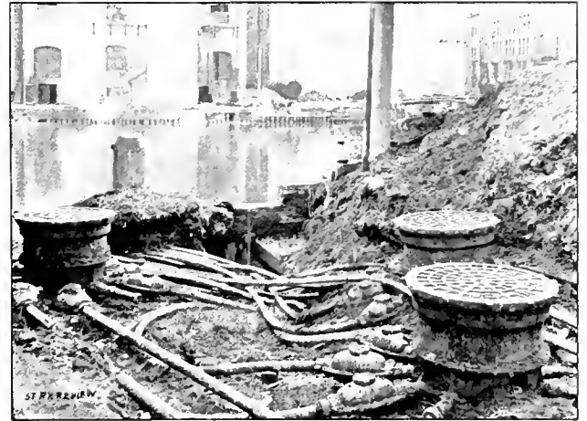
WHERE THE FEEDERS REAPPEAR OPPOSITE THE POWER HOUSE.
