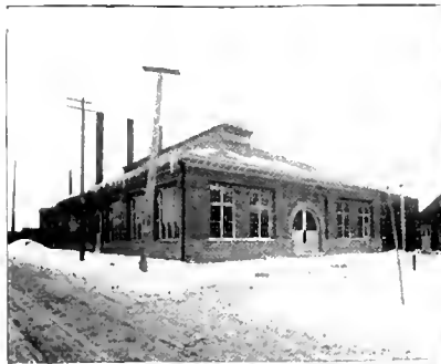
EXTERIOR OF POWER HOUSE.
