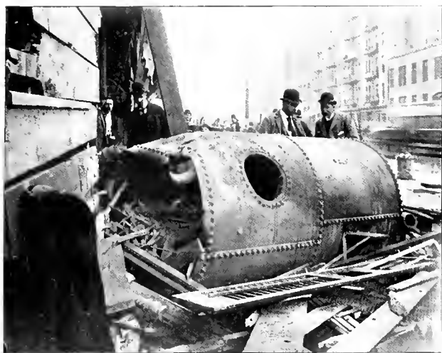
VIEW FROM SIDE OF STREET OPPOSITE CAR BARN, TO WHICH HALF OF BOILER WAS THROWN.
