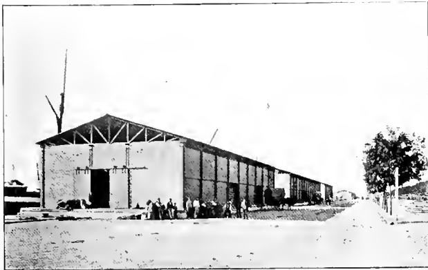
LOADING STATION FOR FREIGHT TRAM CARS.
