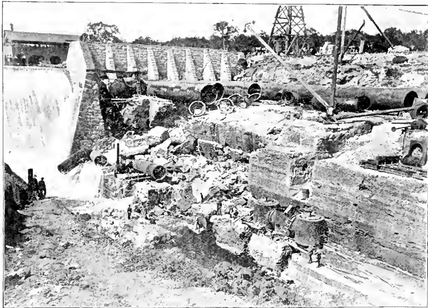
WRECK OF THE AUSTIN DAM.
