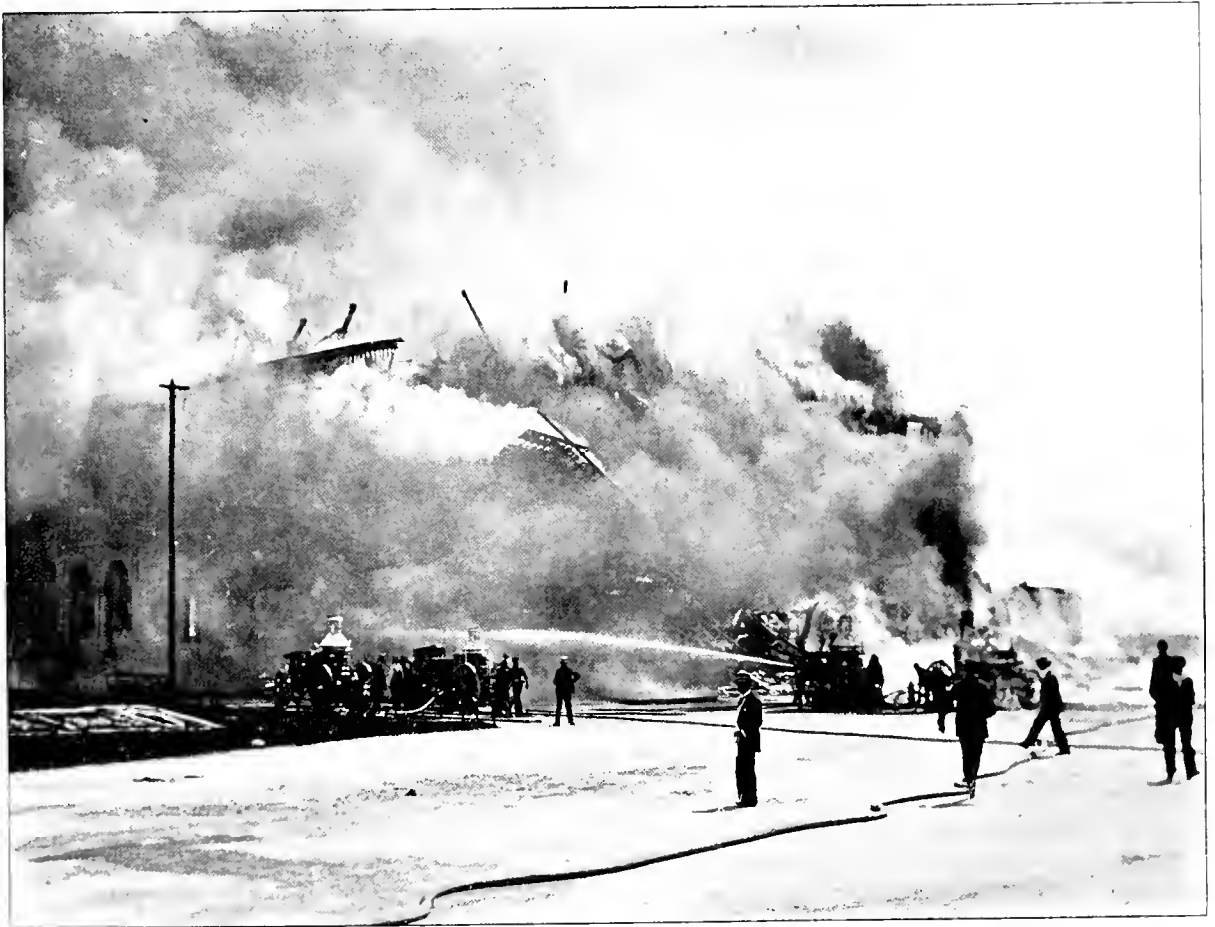
COLD STORAGE FIRE—INSTANTANEOUS PHOTOGRAPH AT INSTANT WHEN TOWER FELL.
