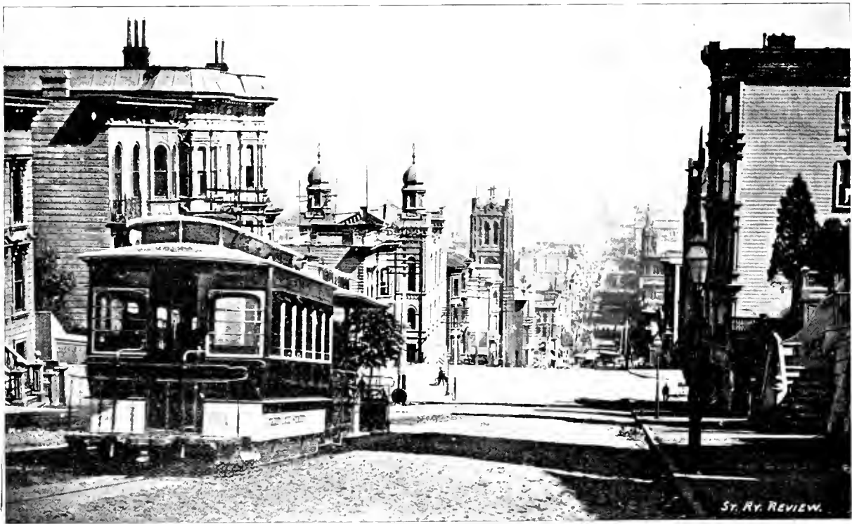
LOOKING DOWN CALIFORNIA STREET, 1893.
