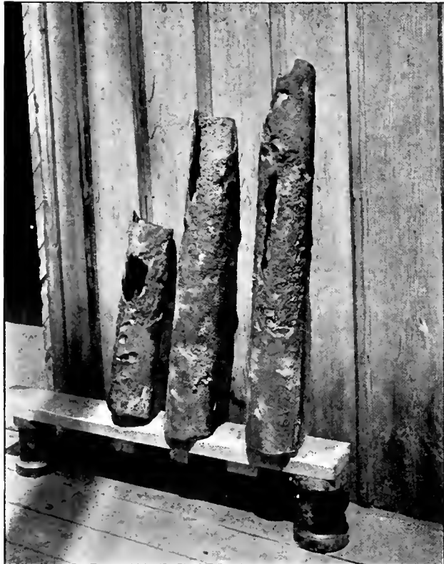
ELECTROLYTIC ACTION AT MILWAUKEE—IRON WATER MAINS.
