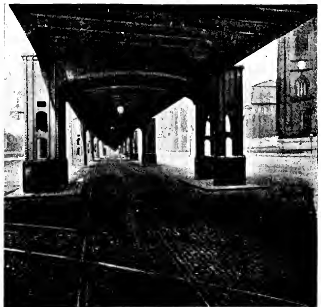
UNDER VIEW OF STRUCTURE.
