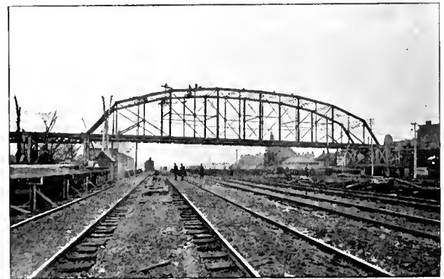
"THE SPAN IS 229 FEET LONG."
