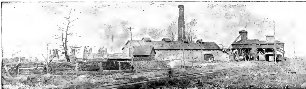
THE POWER STATION AT EDINBURG, ILL.
