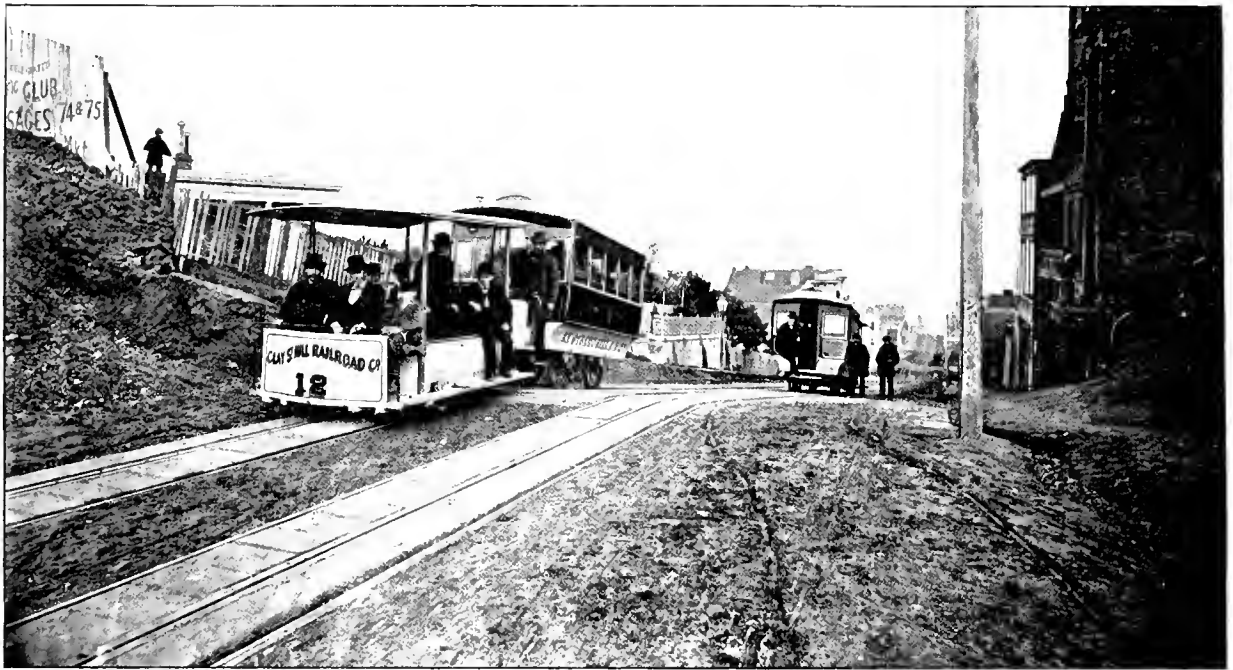
THE FIRST CABLE TRAIN—TAKEN A FEW DAYS AFTER THE OPENING OF THE ROAD.
