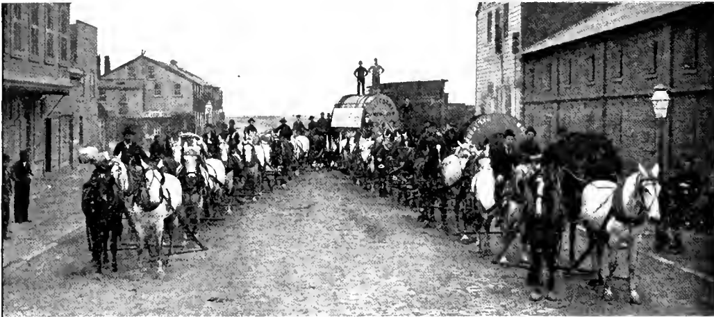
FORTY TONS OF CABLE.
