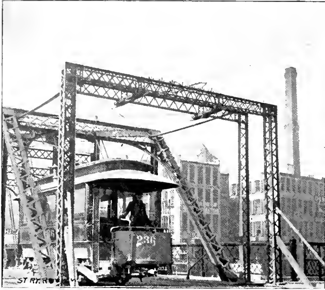
MICHIGAN STREET BRIDGE APPROACH.
