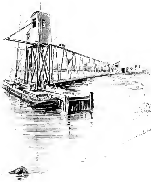
COAL HOIST AND TRAMWAY.
