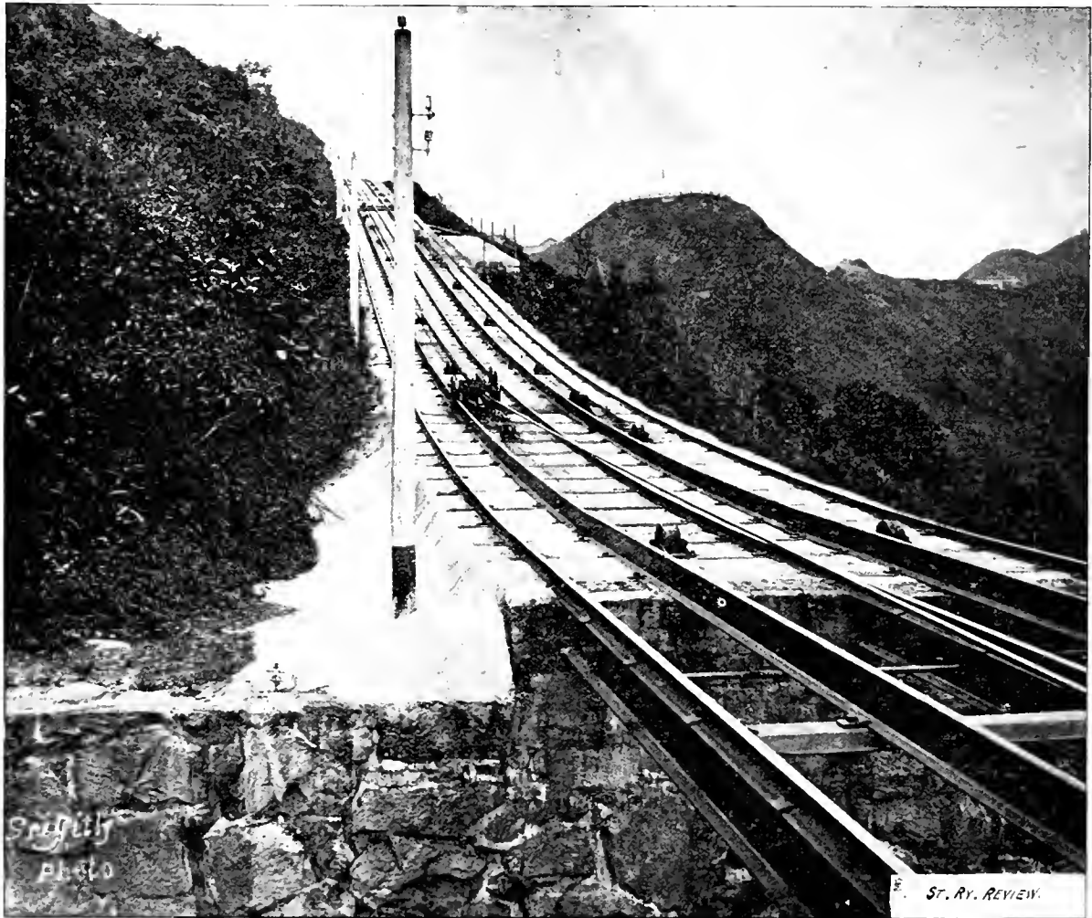
HONG KONG CABLE RAILWAY—SHOWING DEPRESSION PULLEY.
