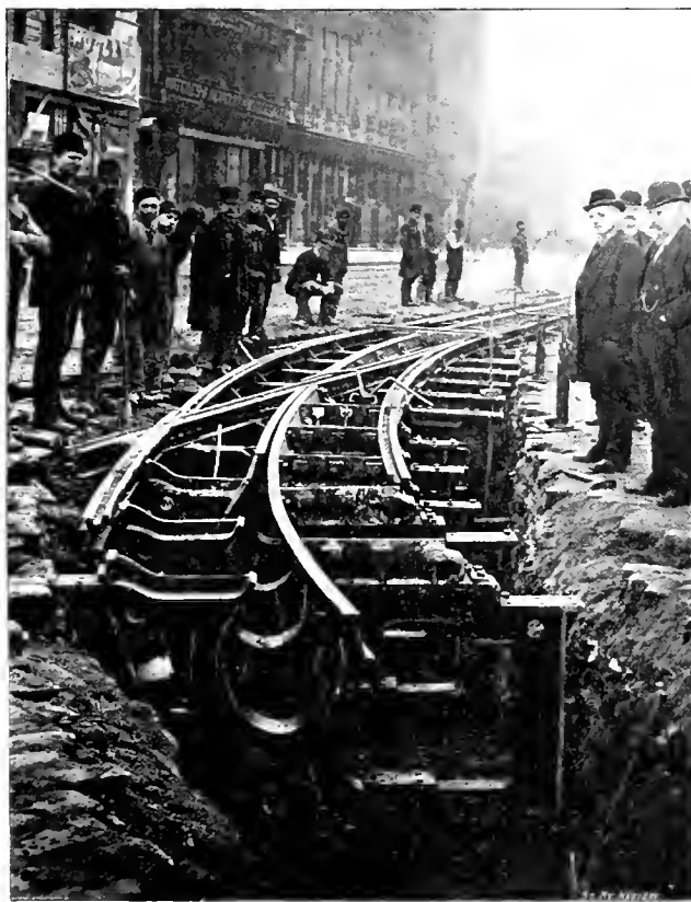
CURVE CONSTRUCTION, STATE AND WASHINGTON STREETS—WEST CHICAGO STREET RAILROAD.
