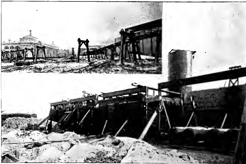
ELEVATED STRUCTURE; POWER HOUSE UNDER CONSTRUCTION.
