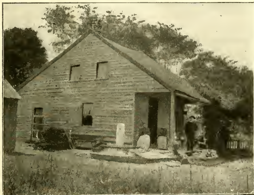
A Type of the Old Houses in Prairie du Rocher. Father C. J. Eschmann, the Parish Priest, is seen on the porch.
