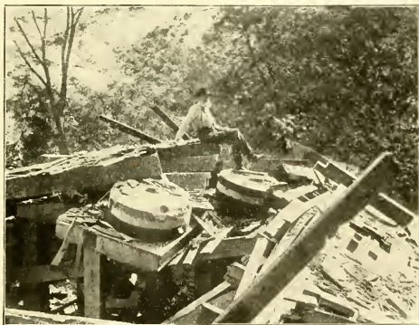
Ruins of a Grist Steam Mill built by the side of the Pax Pagi Mill near Kaskaskia. The two buhr-stones seen in the ruins were brought from France and used in the Pax Pagi Mill. Many of the timbers seen are as much as twelve inches square.
