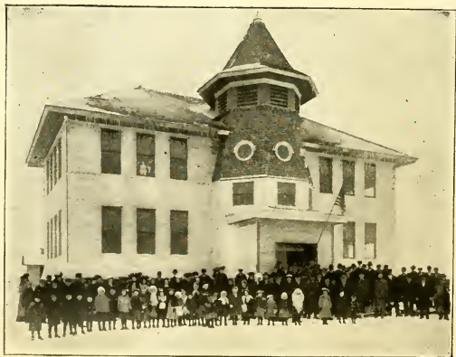
First Consolidated School Building in Illinois. It is located at Seward, Winnebago County, and is the result of the efforts of County Superintendent O. J. Kern.
