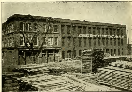
The Building used as a Hospital in Mound City, to which were brought the Wounded Soldiers from the Battlefield of Pittsburg Landing.
