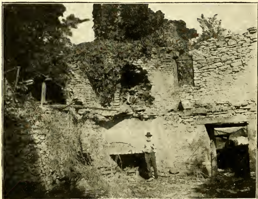
A View of the Ruins of a Gristmill a mile northeast of Kaskaskia. The Mill was built by one Pax Pagi early in the Eighteenth Century. It was run by water power. In this mill was ground the wheat and corn which furnished food for the French Soldiers stationed at Fort Duquesne in the French and Indian War. Pax Pagi and his negro slaves were massacred by Kickapoo Indians, their bodies chopped to pieces and thrown into the grain hoppers. It was operated till 1855. The picture shows the basement room.
