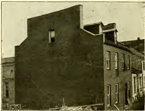
The Rawlings House in Shawneetown, where LaFayette was tendered a Reception and Banquet. The building burned recently.
