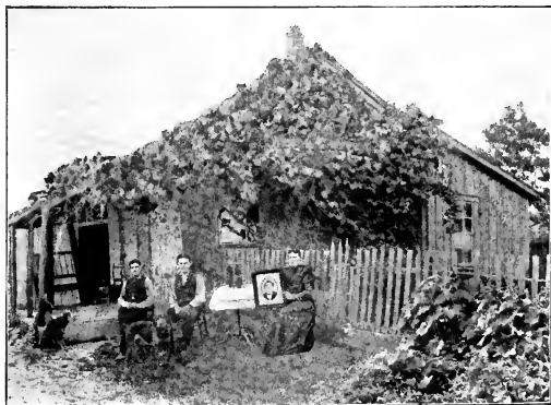
A Mud House. This house was built of clay mixed with straw. It was built in 1852 and stood fifty years. It stood at the south edge of Richland county and is one of many such houses built in the southeastern part of the state in an early day.
