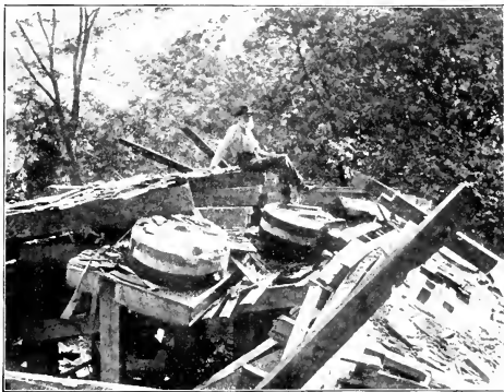
Ruins of a Grist Steam Mill built by the side of the Pax Pagi Mill near Kaskaskia. The two buhr-stones seen in the ruins were brought from France and used in the Pax Pagi Mill. Many of the timbers seen are as much as twelve inches square.
