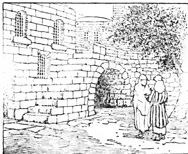
Outside Stairs to the Roof.
