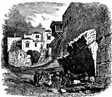
Remains of Arch of Bridge of the Temple. (See p 73.)
