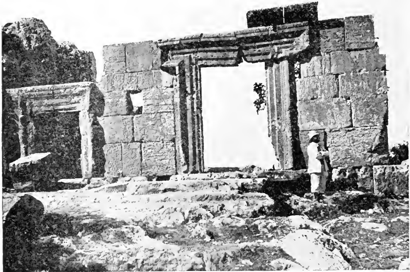
SOUTHERN FAÇADE OF SYNAGOGUE AT MERON—UPPER GALILEE
