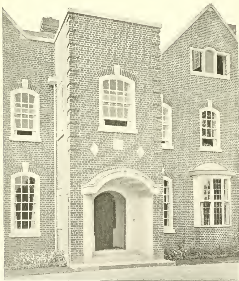
RED COURT, HASLEMERE: ENTRANCE PORCH
