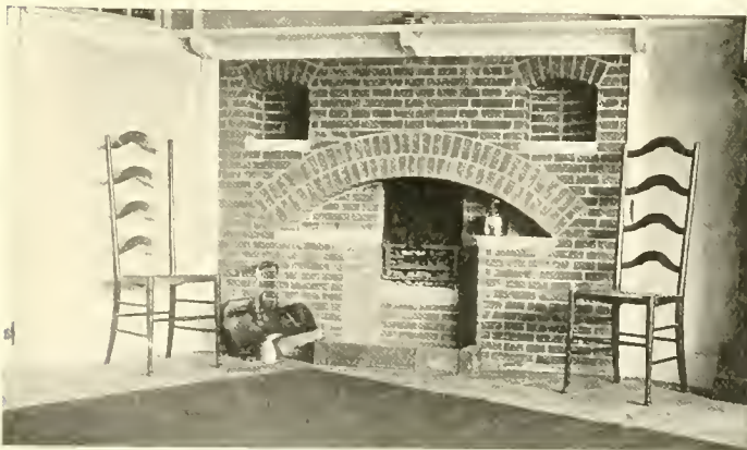
FIREPLACE IN THE HOUSE AT FRENHAM C. F. A. VOYSEY, ARCHITECT
