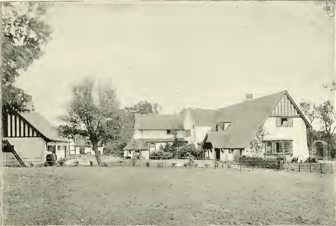
HOUSE AT CASTLE MORTON, WORCESTERSHIRE
