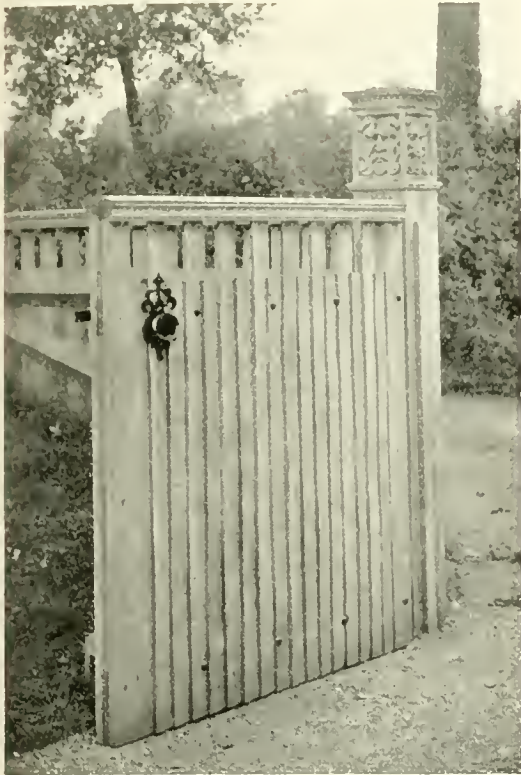
ENTRANCE GATE TO DRIVE AT BOWDEN GREEN
