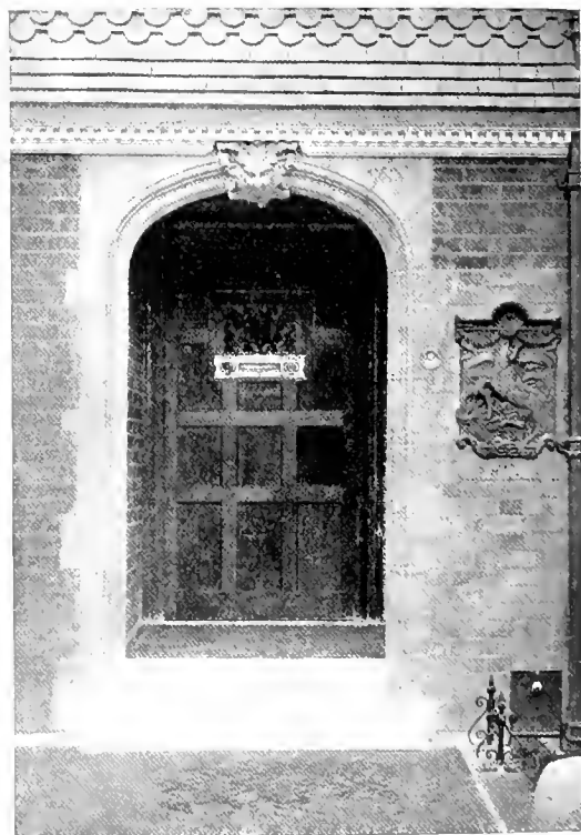
THE FRONT DOOR — ARNOLD MITCHELL, ARCHITECT
