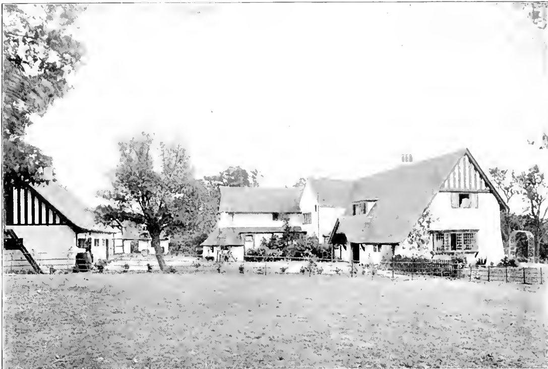
HOUSE AT CASTLE MORTON, WORCESTERSHIRE
