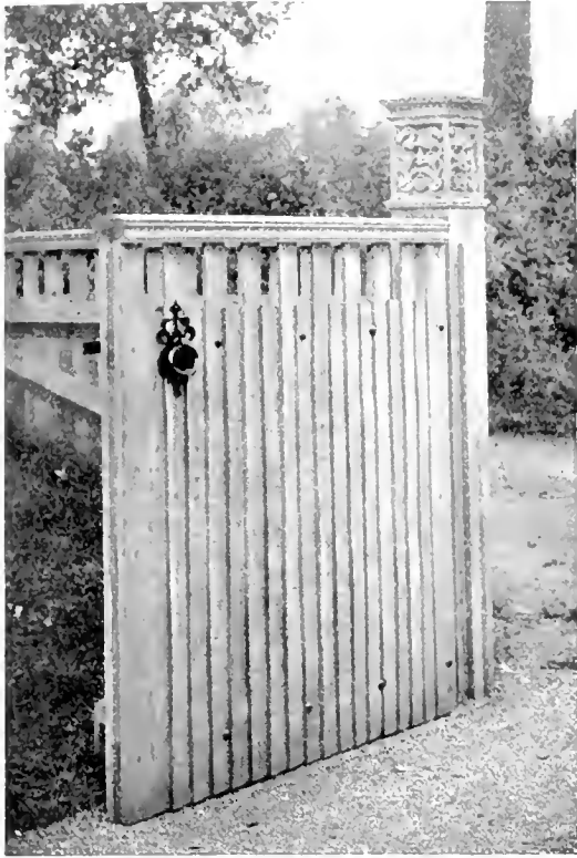
ENTRANCE GATE TO DRIVE AT BOWDEN GREEN
