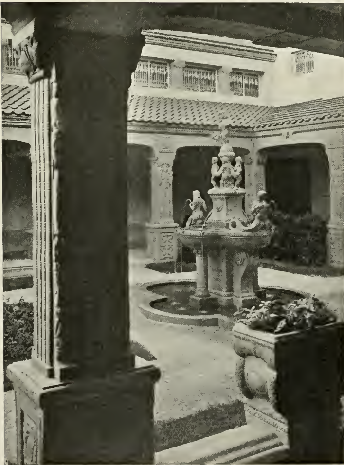
FOUNTAIN COURT AT HESSIAN NATIONAL EXHIBITION, DARMSTADT GENERAL DESIGN BY BAUINSPEKTOR JOST, BAD NAUHEIM. PLASTIC DECORATION AND FOUNTAIN FIGURES BY H. JOBST. TERRA-COTTA WORK EXECUTED BY GROSSHERZOGICHE KERAMISCHE MANUFAKTUR, DARMSTADT
