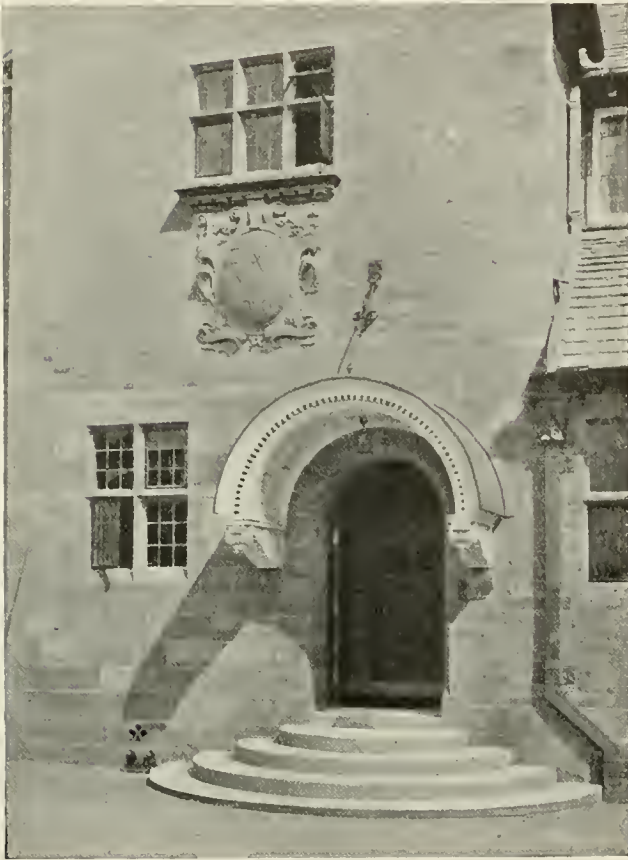
MAIN ENTRANCE TO MR. AGNEW'S HOUSE AT WARFORD PERCY WORTHINGTON, ARCHITECT
