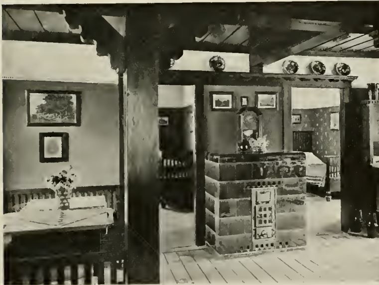
INTERIOR OF ARTISAN'S COTTAGE SHOWING LIVING ROOM WITH STOVE FOR HEATING THREE ROOMS GEORG METZENDORF, ARCHITECT
