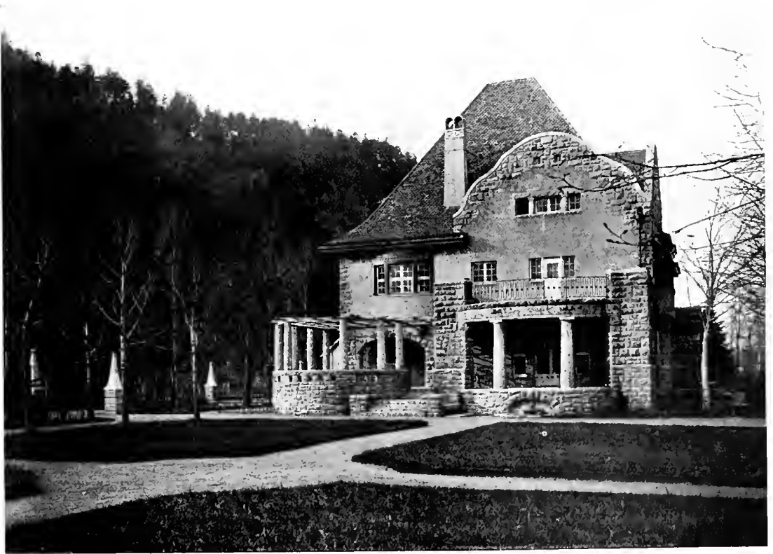
"OSTMÄRKER HOF," GUTACH, BREISGAU, GERMANY
