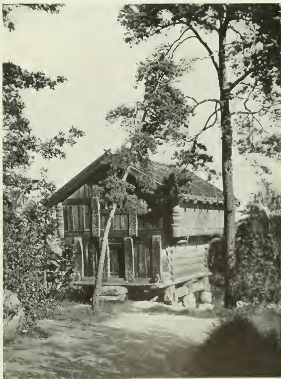
OPEN-AIR MUSEUM, SKANSEN, SWEDEN. THE VASTVELL STOREHOUSE
