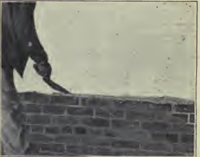
Fig. 37.—Working right to left.—Spreading mortar on the interior face tier.
