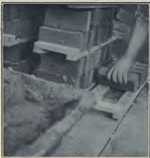
Fig. 7. — Wrong way to pick up brick from the lower tier on the packet.
