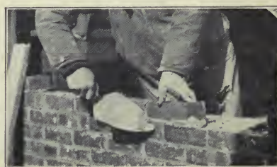
Fig. 27. — Cutting off the mortar after the brick is laid on the exterior face tier.
