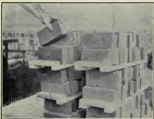
Fig. 4.—Right way to pick up brick from upper tier on the packet.
