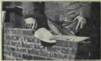
Fig. 25. — Cutting off mortar before the brick is laid on exterior face tier.
