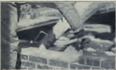
Fig. 28. — Throwing mortar on interior face tier.
