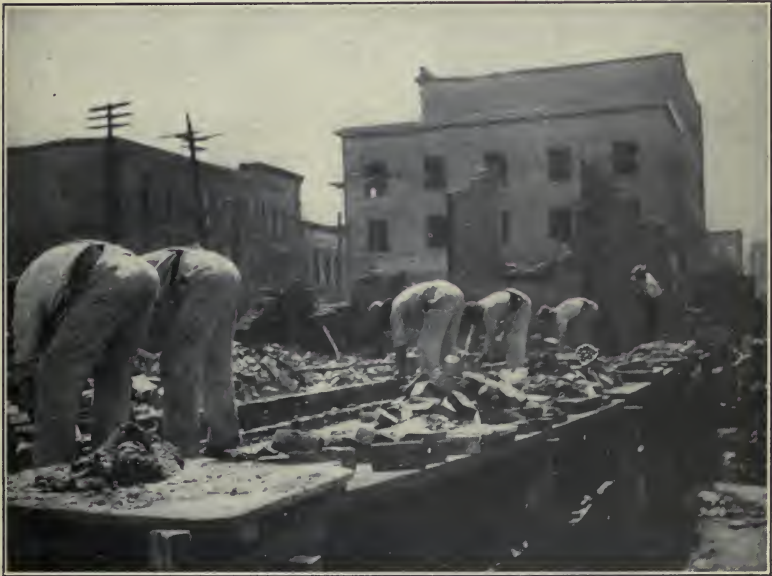
Fig. 23. — Common type of Trestle Horse Staging. Bricklayers cannot be expected to lay as many brick per day when working in this position as when standing up between a wall and a stock platform, each 2 ft. high.
