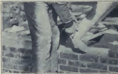
Fig. 29. — Spreading mortar on interior face tier.
