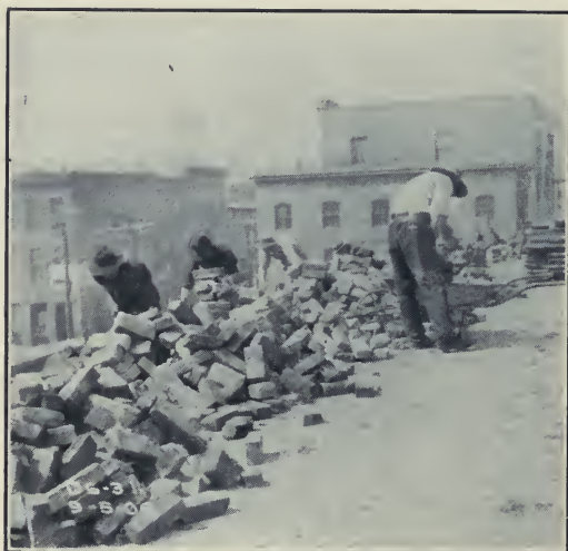
Fig. 9.—The usual method of providing the bricklayer with material.
