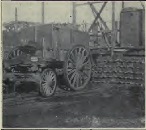
Fig. 17.—Two-horse carts with horses changed from the empty to the full carts will require fewer and cheaper motions than any other methods of transportation.
