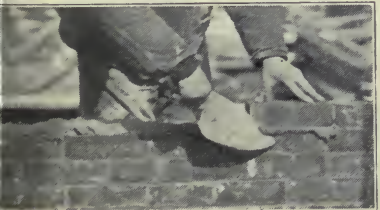
Fig. 38.—Working left to right.—Cutting off mortar after brick is laid on exterior face tier.
