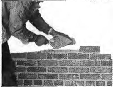
Fig. 42.—Working right to left.—Buttering right-hand end of brick in hand to be laid on interior face tier.
