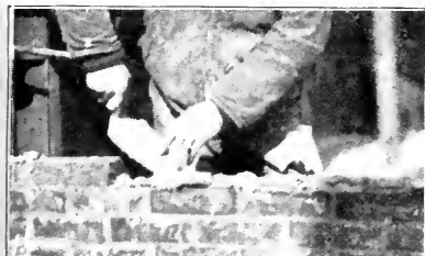
Fig. 34.—Working right to left.—Spreading mortar on exterior face tier.
