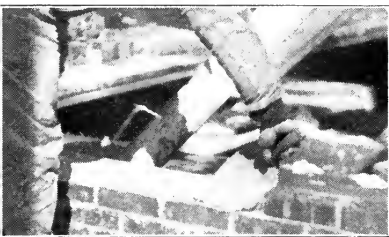
Fig. 28. — Throwing mortar on interior face tier.
