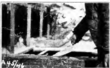
Fig. 39.—Working left to right.—Spreading mortar on the interior face tier.
