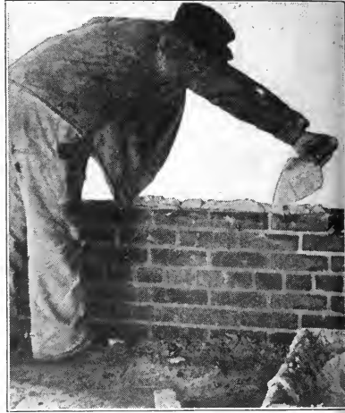
Fig. 41.—Working left to right.—Throwing mortar on the interior face tier.
