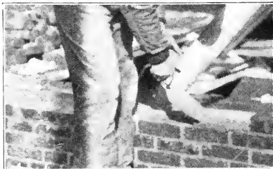
Fig. 29. — Spreading mortar on interior face tier.
