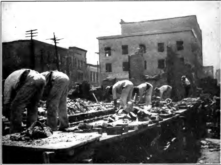
Fig. 23. — Common type of Trestle Horse Staging. Bricklayers cannot be expected to lay as many brick per day when working in this position as when standing up between a wall and a stock platform, each 2 ft. high.
