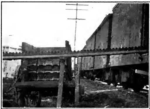
Fig. 18. — Loading carts with 90-pound packs of brick fed on gravity conveyors.
