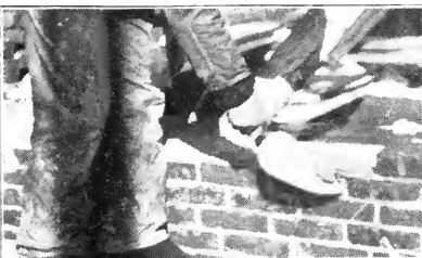
Fig. 30. — Cutting off mortar before brick is laid.
