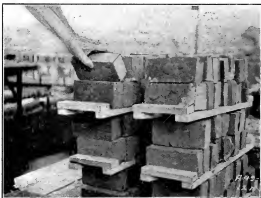
Fig. 5.—Wrong way to pick up brick from upper tier on the packet.
