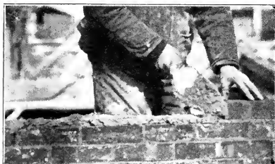
Fig. 35.—Working left to right.—Buttering end of laid brick on exterior face tier.
