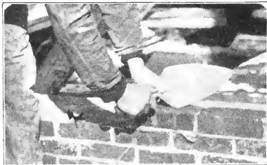
Fig. 31. — Tapping down brick after laying on interior face tier.
