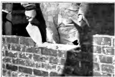
Fig. 24. — Spreading mortar on exterior face tier.
