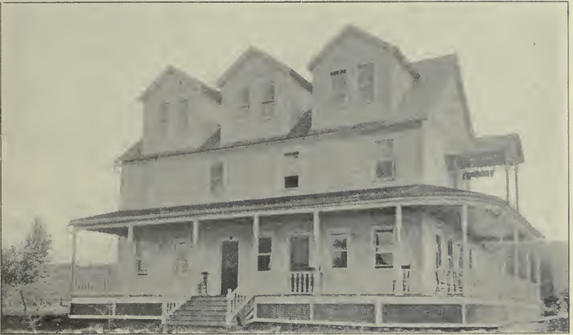
NEWER TYPE OF BOARDING HOUSE. WINDOWS ARE NARROW, AND THERE ARE TWO BEDS IN A ROOM. MANY OF THIS TYPE ARE ADVERTISED AS "MODERN" AND HAVE FLUSH TOILETS ON THE SECOND AND THIRD FLOORS, GENERALLY IN A RATIO OF ONE TO TWENTY OR MORE GUESTS AND RARELY CLEAN
