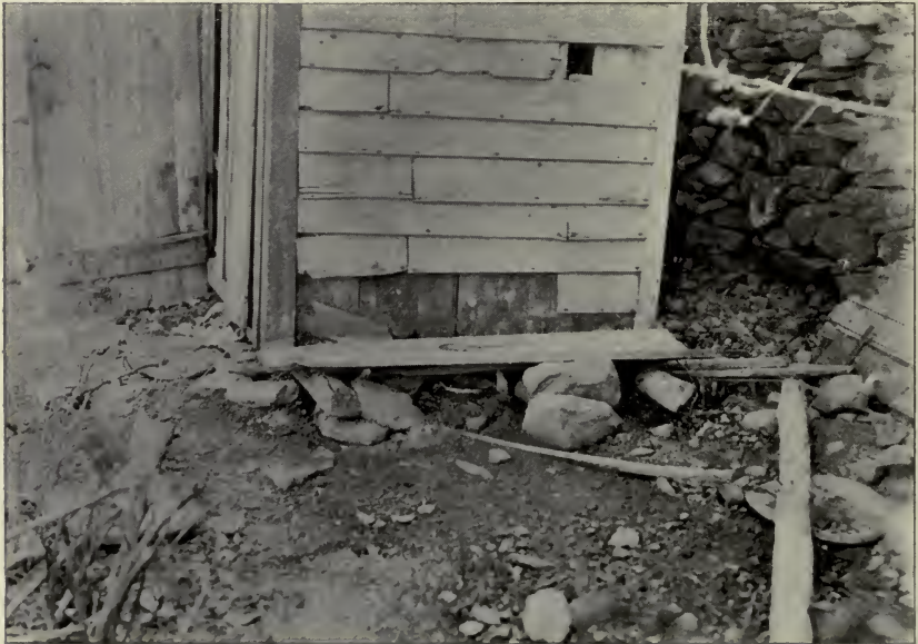
PRIVY SET ON TOP OF GROUND. NO REMOVAL BOX OR PAILS. FECAL MATTER OVERFLOWING ON GROUND OUTSIDE, SATURATION FOR FOUR FEET. USED BY AT LEAST 24 PERSONS ALL SEASON
