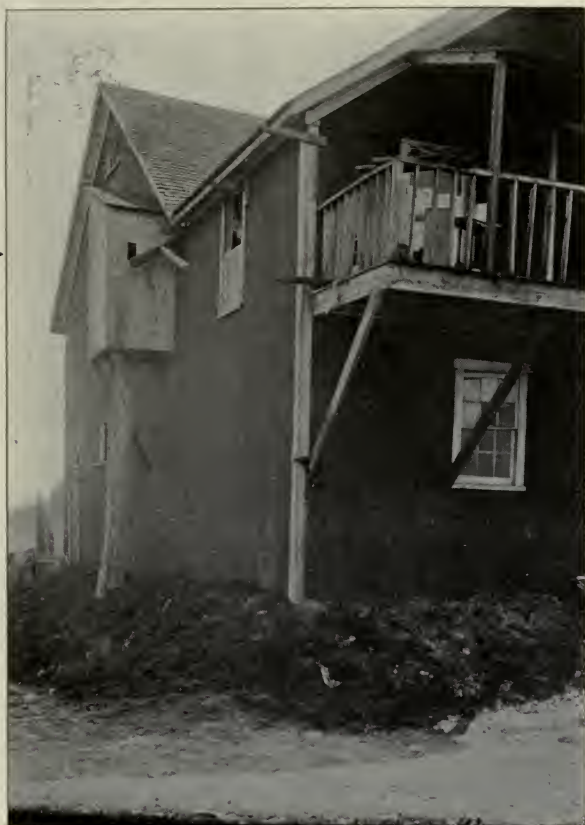
FOUR BEDROOMS WITH THIN WALLS, AND ACCESS THROUGH, HAVE BEEN PARTITIONED OFF IN LOFT OF BARN FOR USE OF FAMILY AND HELP. PRIVY WITH SHAFT ENDING AT GROUND (NO VAULT) CONSTRUCTED ON SIDE OF BARN. ENTRANCE THROUGH BEDROOM
