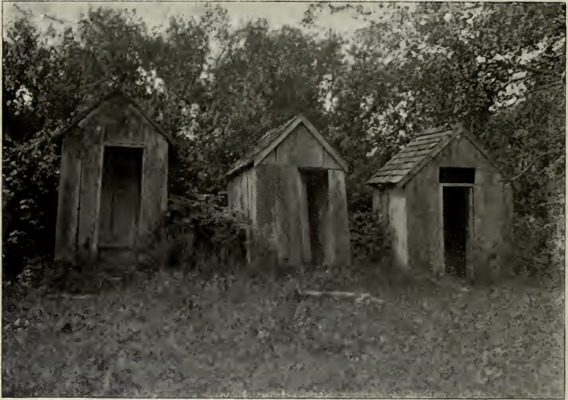
UNUSUAL EQUIPMENT OF PRIVIES. GENERALLY ONLY ONE. SHELTERS RICKETY, FLOORS ROTTEN, SEATS FILTHY
