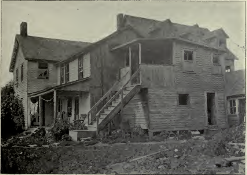
FLIMSY CONSTRUCTION OF ADDITIONS; BACK YARD GARBAGE STREWN AND SATURATED WITH SLOPS
