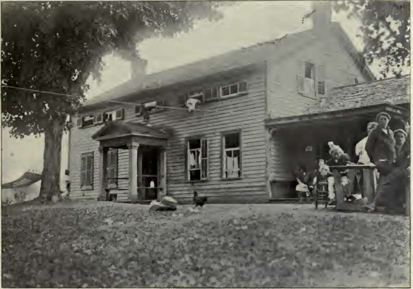
TEN BEDROOMS. ONE FAMILY IN EACH, WITH COMMON KITCHEN AND DINING ROOM; 15 TO 20 ADULTS; 30 TO 40 CHILDREN. WATER SUPPLY, A SPRING WHICH RECEIVES SURFACE DRAINAGE AND WASTE FROM KITCHEN SINK; ONE PRIVY WITH LOOSELY BUILT REMOVAL DRAWER, OVERFLOWING AT TIME OF INSPECTION
