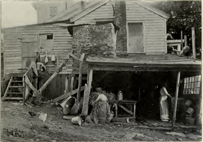
KITCHEN AND DINING ROOMS IN ONE-STORY EXTENSION WITH SEVERAL ADDITIONS. LAUNDRY AND PART OF PREPARATION OF VEGETABLES, DRESSING OF CHICKENS DONE UNDER SHED. NOTE LARGE BAKE OVEN SUPPORTED ON POSTS
