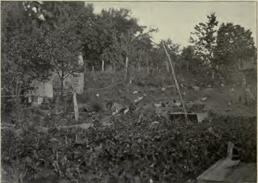
SIDE YARD DIRTY AND UNKEMPT. TWO PRIVIES AT LEFT OF PICTURE, VAULTS FULL, SUPPORTS ROTTED, YARD SLOPES TOWARD SPRING WHICH IS WATER SUPPLY OF HOUSE
